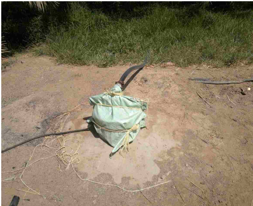
Figure 495: Inappropriate cap-seals around wells may allow the entry of pollutants.
