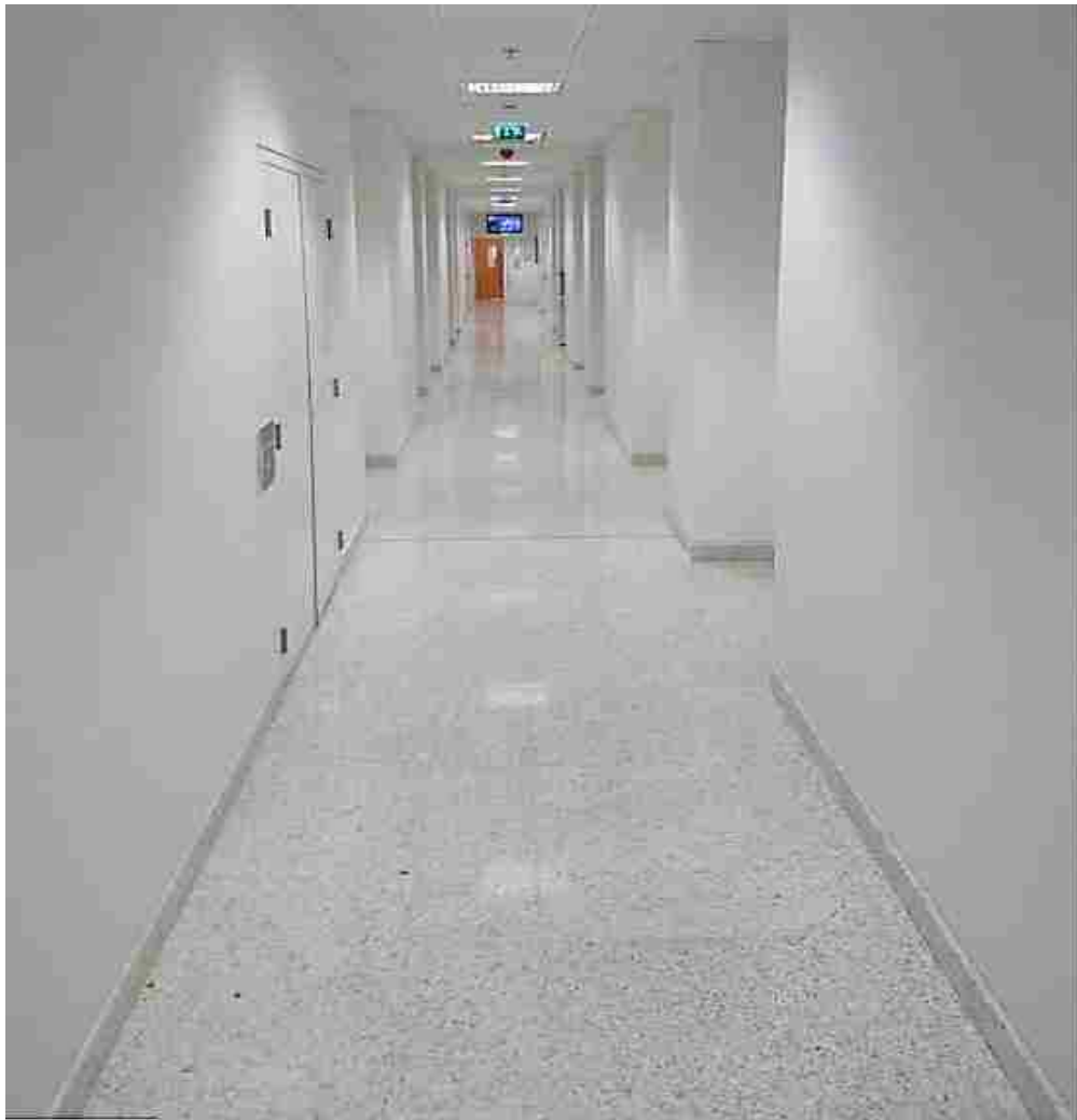
Figure 7: Visual of the central corridor on the 2nd floor of building E4
