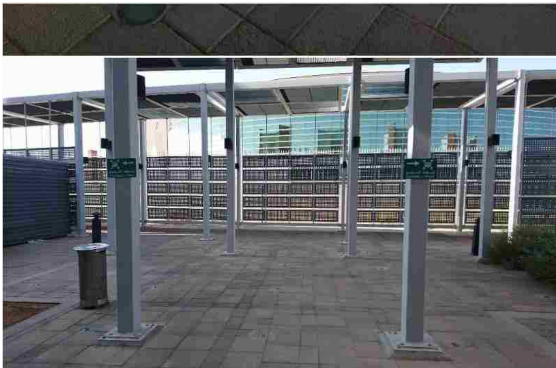
Figure 22: Exit out of the E4-building (female side)
