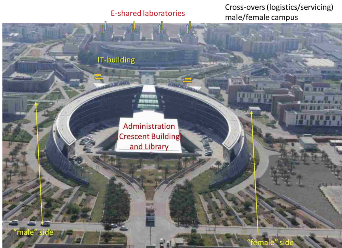
Figure 2: New Maqam campus showing the movement of service personnel possible between the male and female
