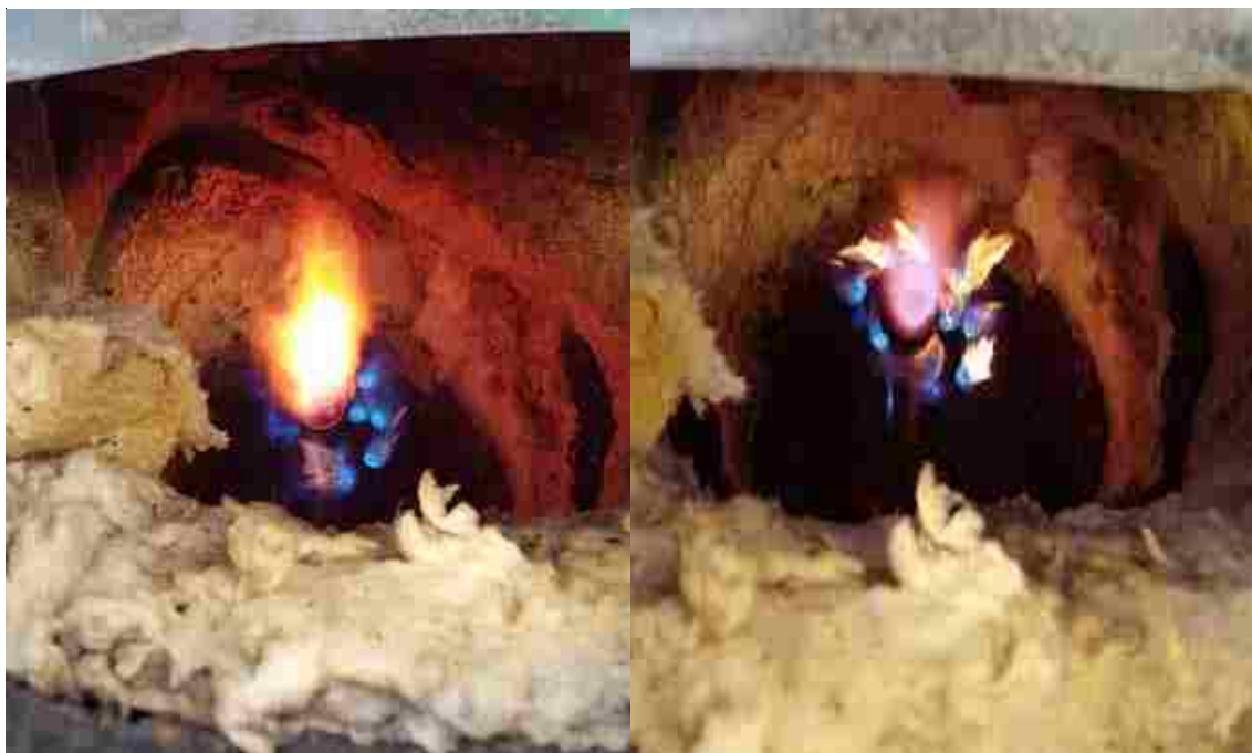
Figure 4.3. Syngas flame in combustion flare a) left less air flow b) high air flow right
