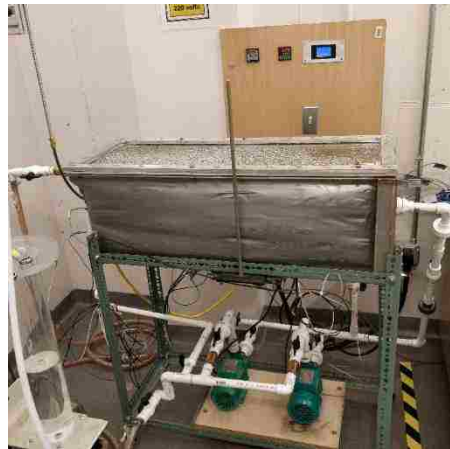
Figure 4. Hot Water System
