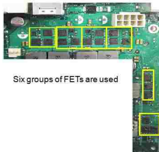
Fig. 1.7 Test structure showing the 6 phases of the converter.
