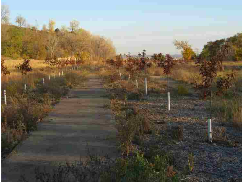
Figure 6.14: Concrete slabs (used for railroad car maintenance) extant at the Vento Sanctuary
