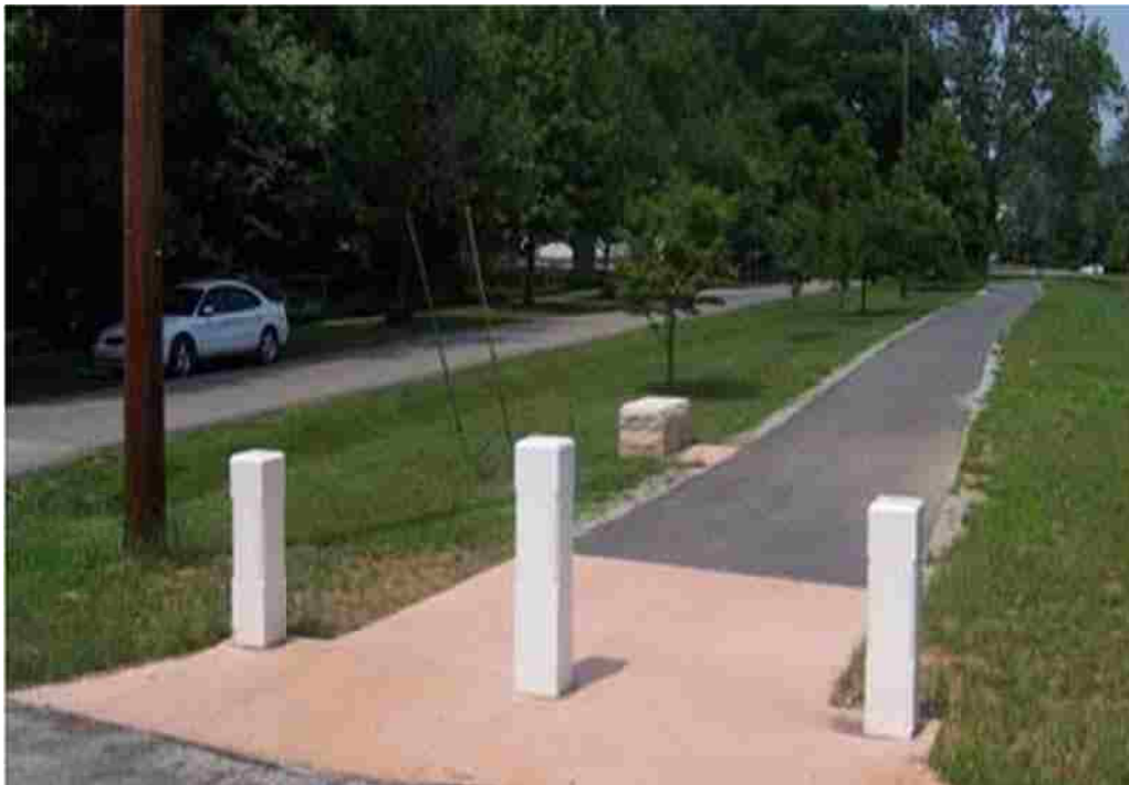
Figure 7.6: Oldham County Greenway on west edge of downtown LaGrange. Photo courtesy of Oldham County Greenways
