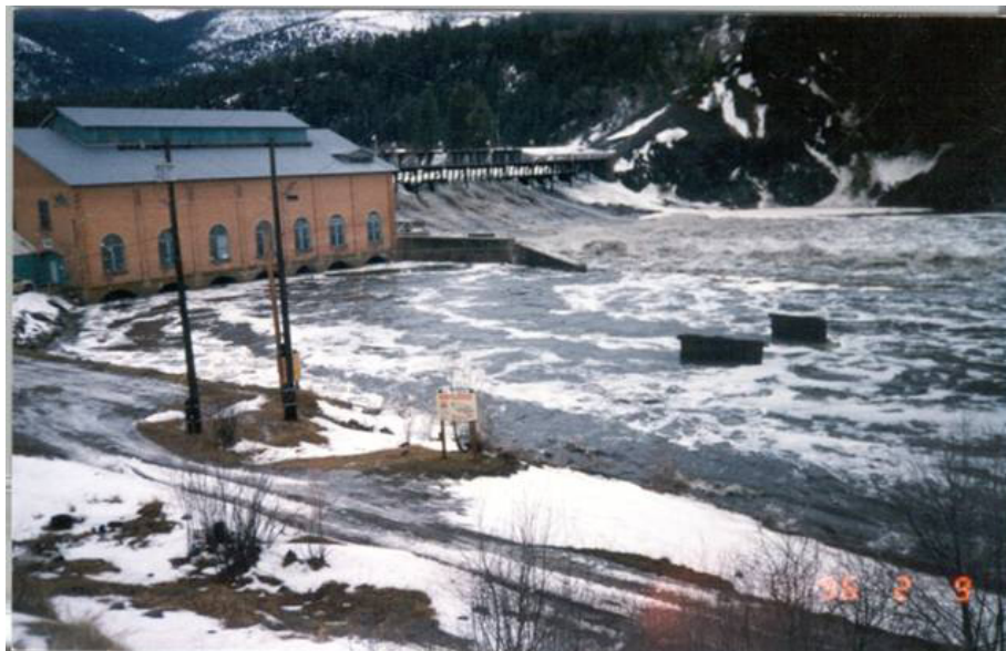
Figure 1.3. The February, 1996 ice event forced the drawdown of Milltown Reservoir to avoid impairing the dam's structure (Source: Judy Martz, Bonner Milltown History Center)
