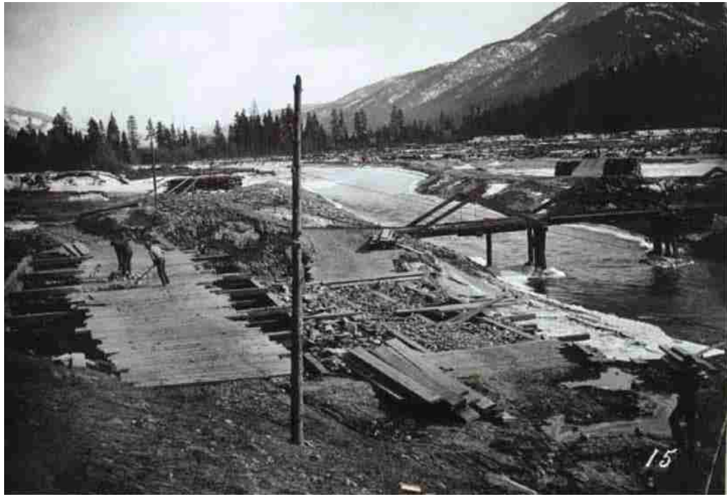
Figure 4.6. Clark Fork River, Looking Upstream, c. 1905. Captured during the early stages of dam construction, this image shows the extent of floodplain forest cleared as well as mature forested areas farther upstream
