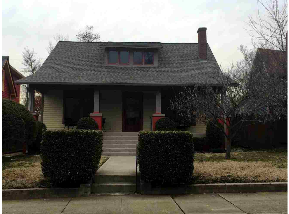
Figure 4.1. A structurally sound bungalow-style home at the junction of Woodland and S. 16th typical of homes in the East End neighborhood and Possible census tract 121.
