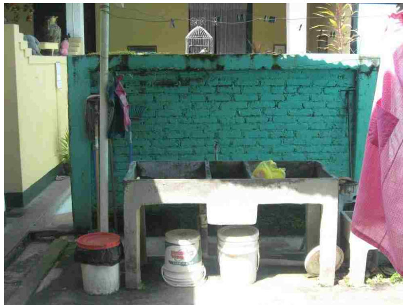
Figure 2.18, A Nicaraguan pila , or sink, used for washing clothes, or sometimes as a kitchen sink.
