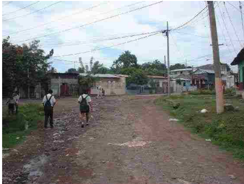
Figure 6.1, Right outside of Granada's historic center, many streets remain unpaved.
