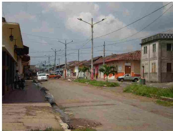
Figure 5.2, Calzada under construction in 2007, but still maintaining its earlier two-way traffic design.
