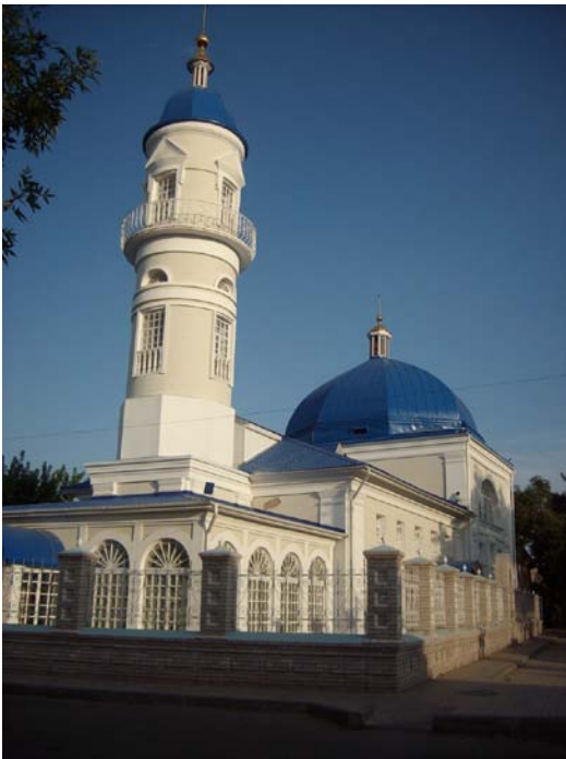
Figure 4.4: White Mosque after renovations.
