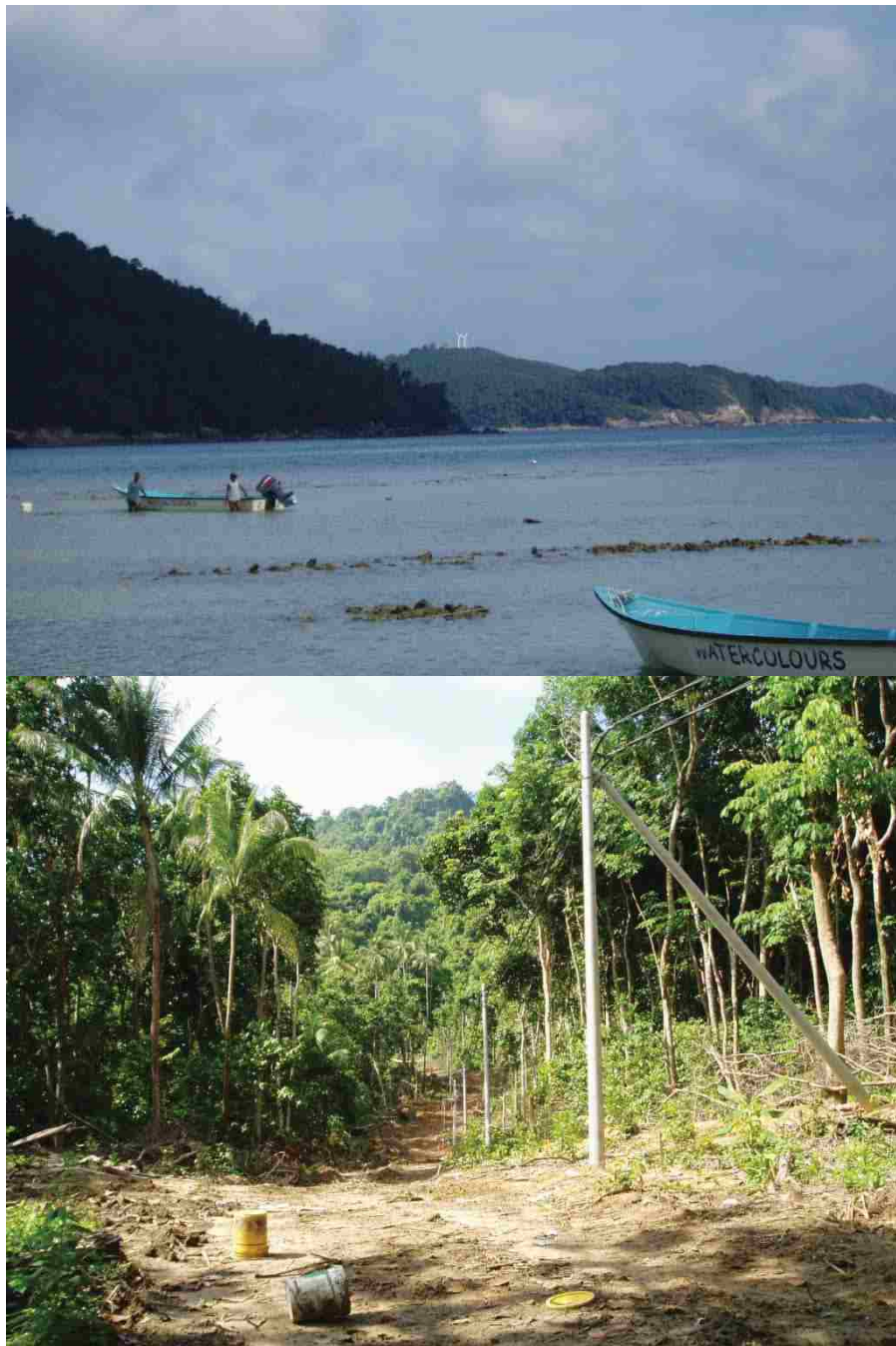
Figure 4.3: Wind turbines and supply lines through the jungle
