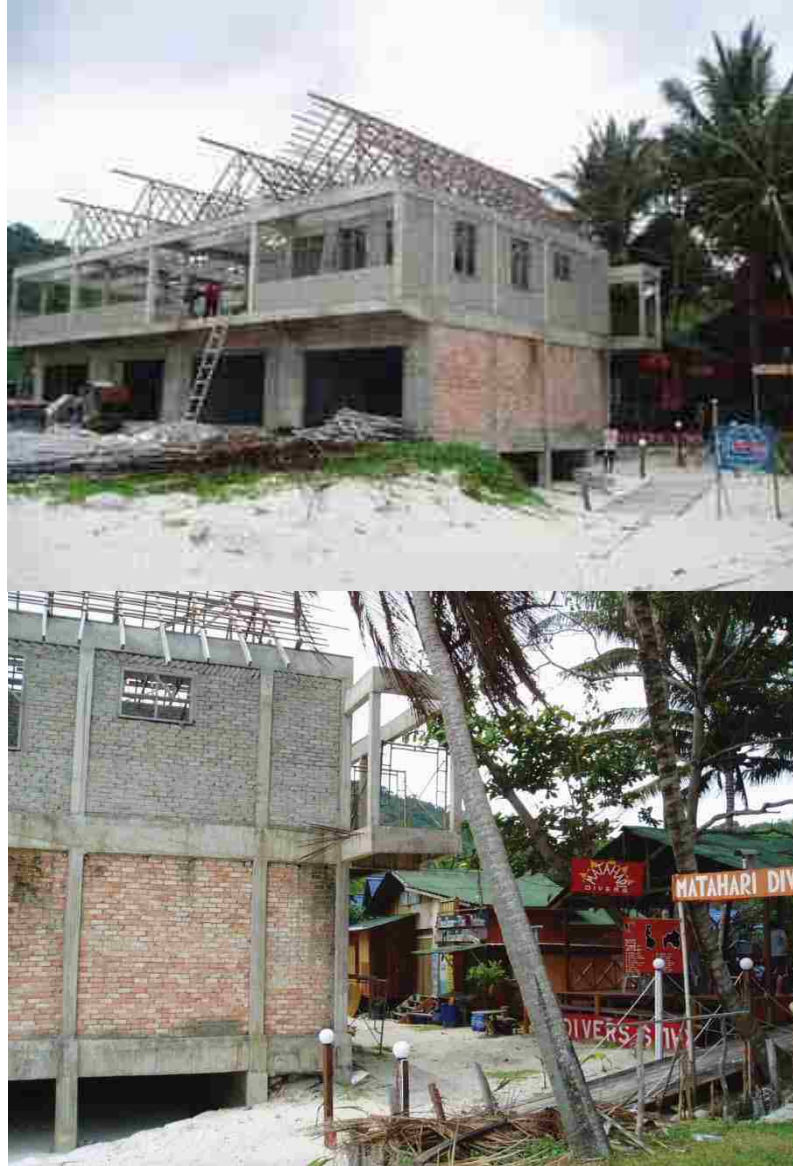
Figure 7.2: Construction of concrete shop in front of existing properties
