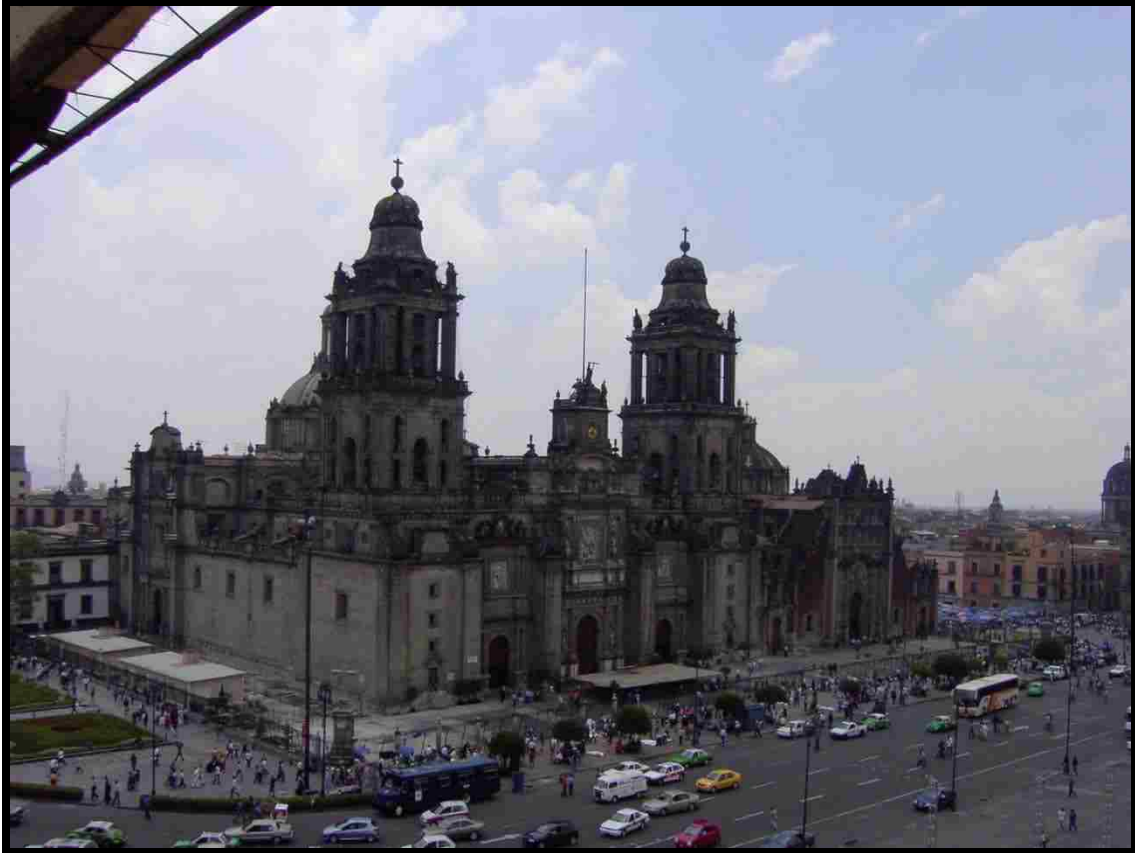
Figure 19. The National Cathedral, located in the Zócalo at the heart of the Centro, is flanked by City Hall and the National Palace. Photo by author
