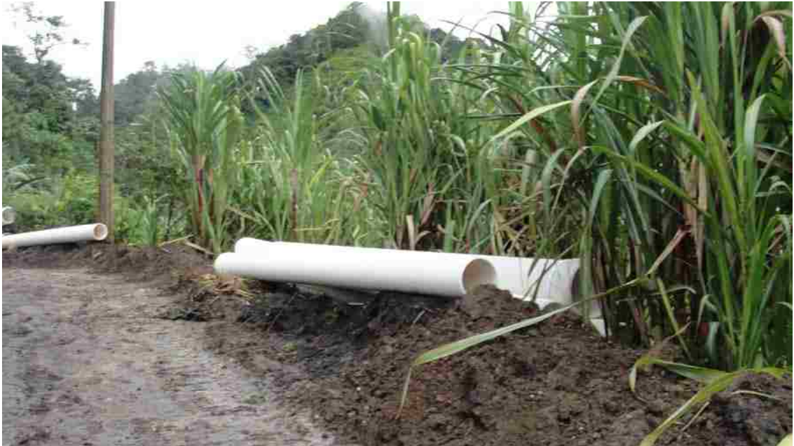
Figure 3.1 Details: Sugar cane crop damage caused by road construction for exploration, Junín community. Photo by author, 2014.
