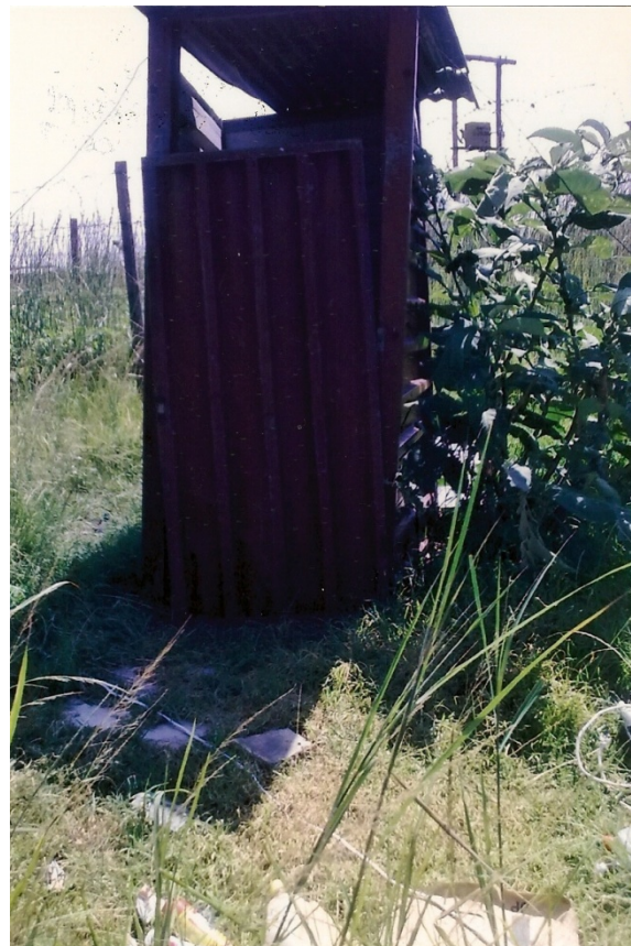
An outdoor toilet. Very unsuitable for a child in a wheelchair.
