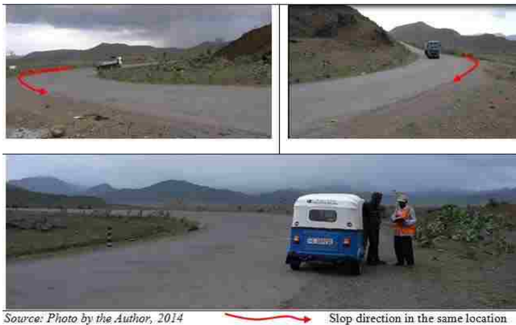
Figure 7. 2: Road Curve with Steep Slopes at Allewuha (11 kms form Hara Town along Corridor 2)
