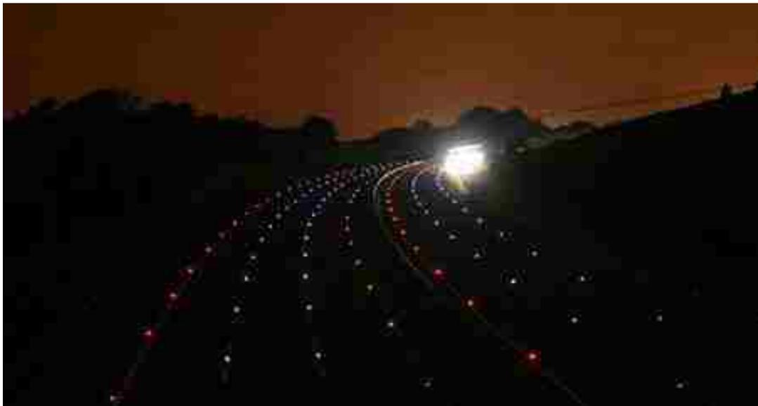
Figure 6.5: Solar-powered road studs in fog (a) and at night (b).
