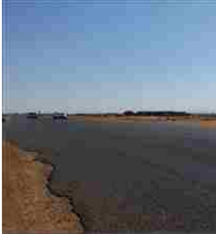
Figure 5.2: Continuous edge-breaks on road P296.
