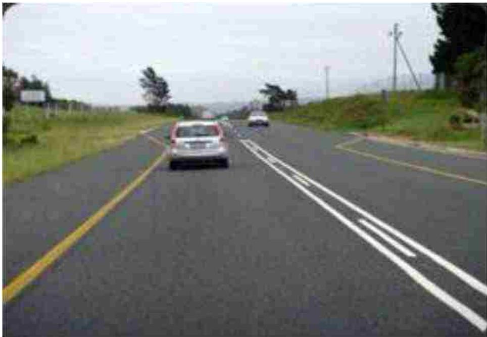
Figure 6.4: Solid lines (a), and barrier and left/right edge lines (b).
