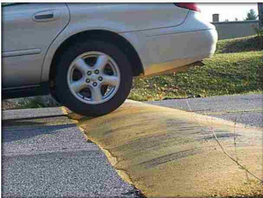
Figure 6.3 a) Temporary speed hump and b) permanent speed hump
