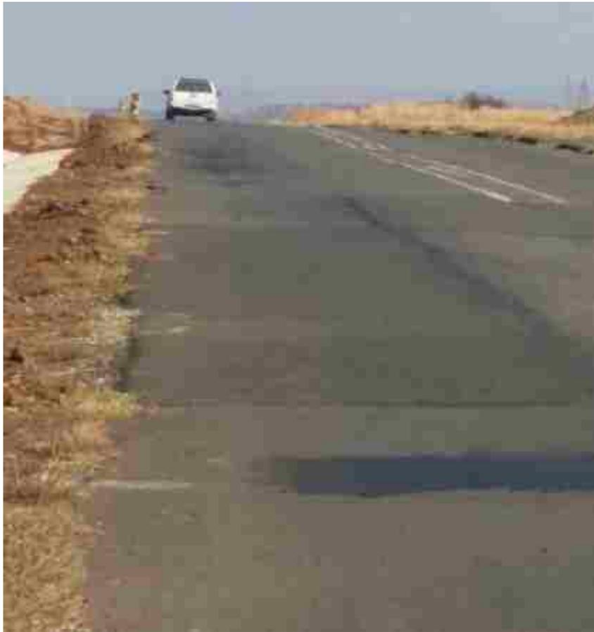
Figure 5.4: Uneven or irregular road surface on road P483.
