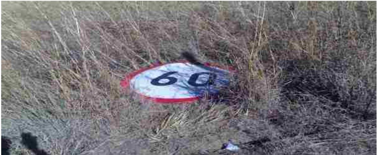
Figure 5.5: Vandalised road sign on road P296.
