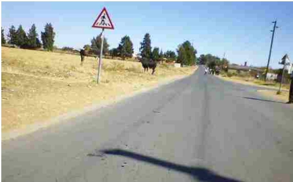
Figure 5.6: Faded and absent road markings on roads P483 (a) and P296 (b).
