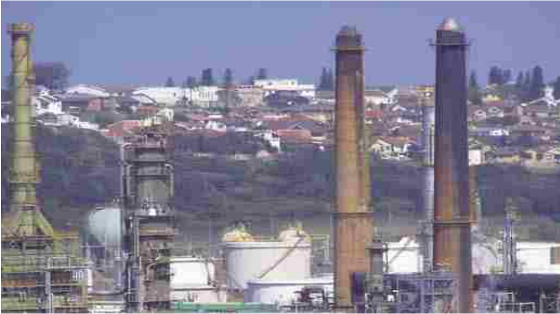
Figure 3.5 Emission stacks in close proximity to Treasure Beach Bluff (DEAT-South Durban Basin MPP Case Study Report: 2007)
