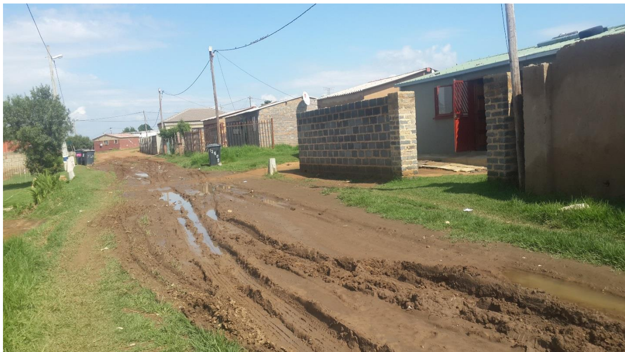
Fig. 5.2 Conditions of the roads in Braamfischerville: Photos by JM Kotane
