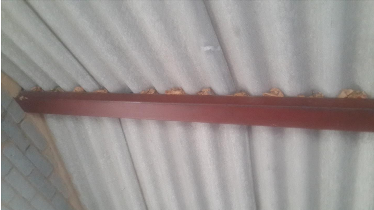
Fig 4.3 Poor building materials- people use paper and other materials to prevent wind and dust from entering the house. Photo by J.M. Kotane
