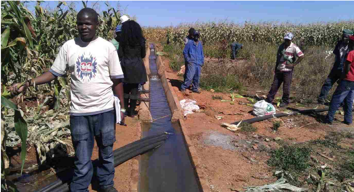
Figure 5.1 Irrigation Expansion underway
