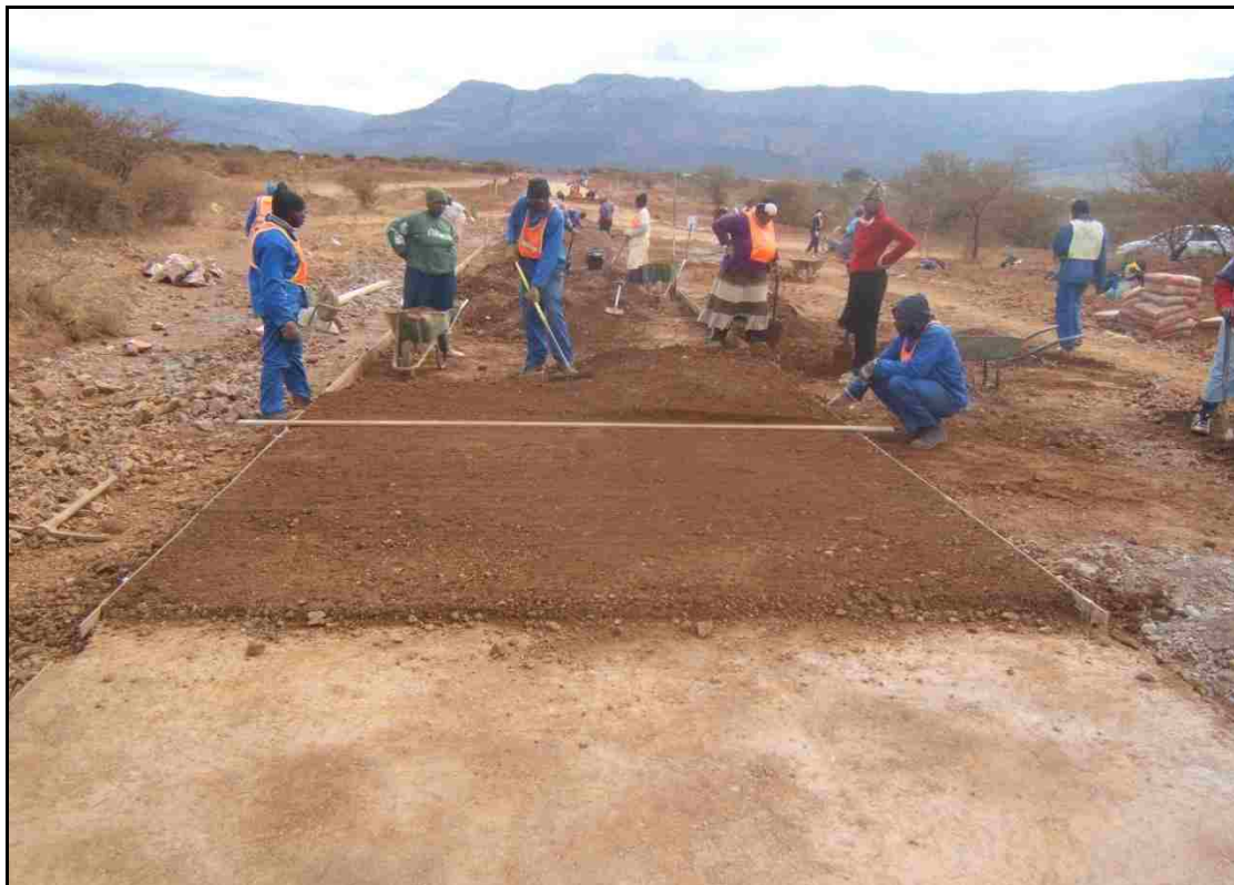
Figure 4.1 (a): Labour-intensive road construction activities
