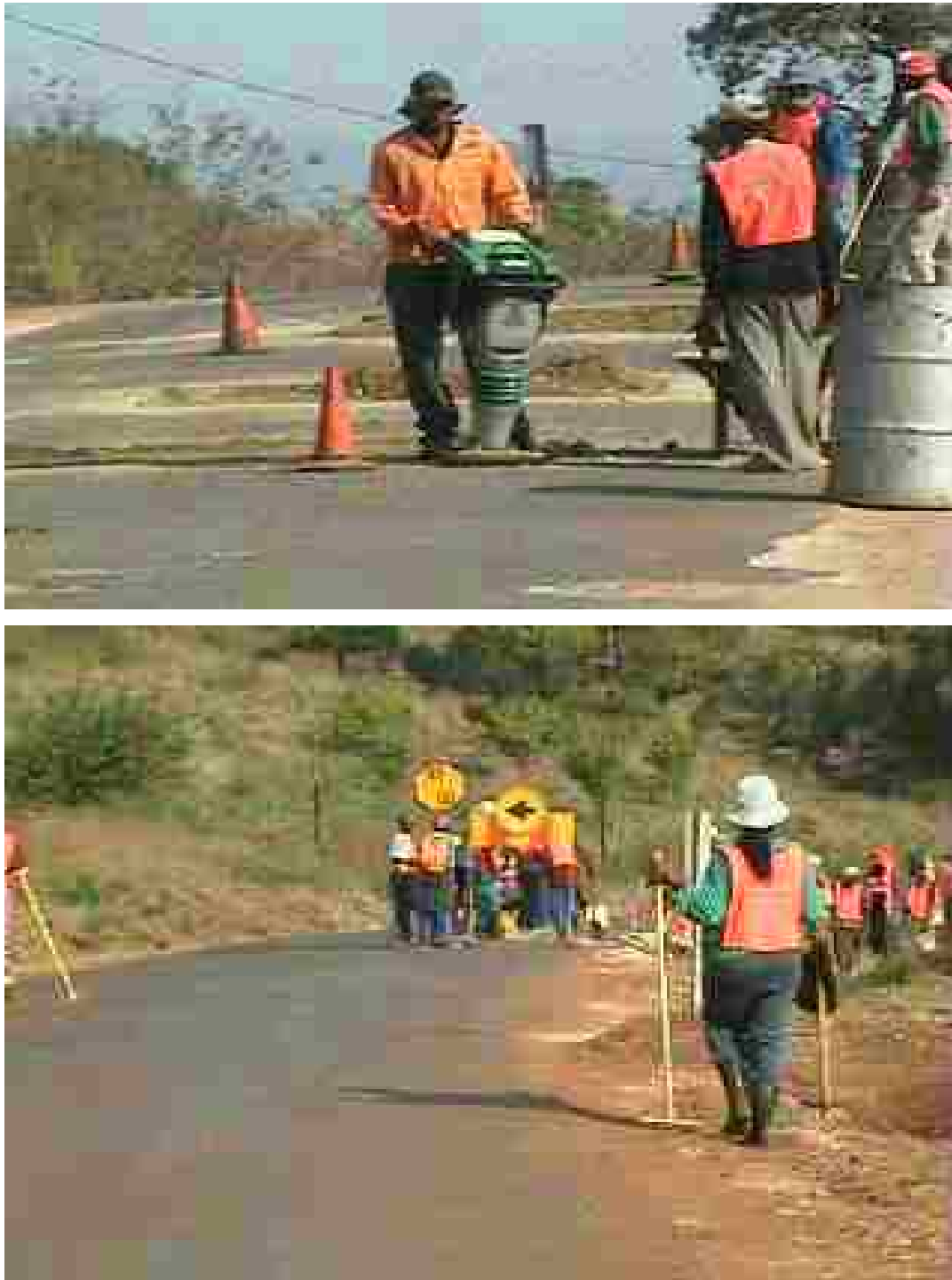
Figure 4.2: Labour-intensive road maintenance activities
