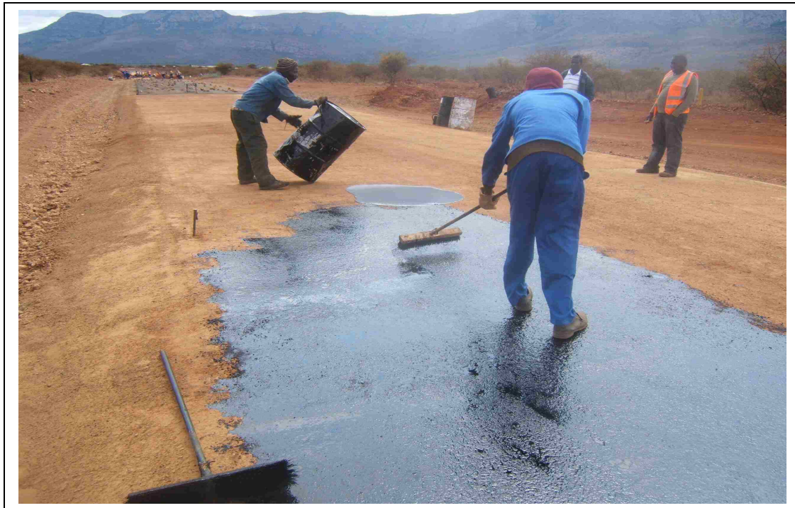
Figure 4.1 (b): Labour-intensive road construction activities
