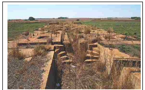
Fig. 8 Ball mill plant foundations.
