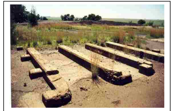
Fig. 2 Part of the concentration plant foundations.
