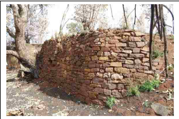
Fig. 13 Dry stone retaining wall in boiler house pit. Reuse of 1890s dressed stone.
