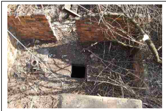
Fig. 1 View looking down onto the shaft cap.
