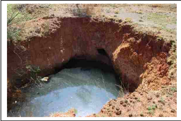
Fig. 9 Collapsed upper stope near winze E2.
