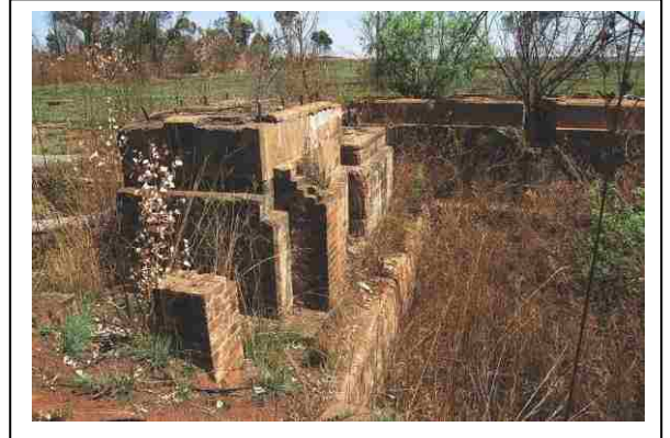
Fig. 10 Part of the boiler plant foundations.
