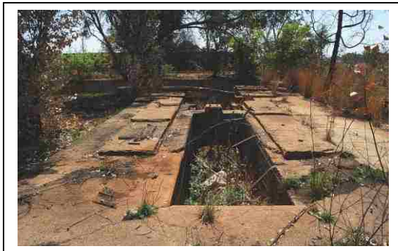
Fig. 3 Boiler plant foundations.
