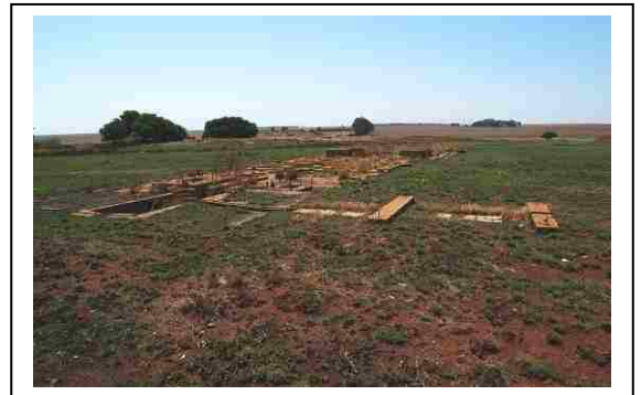
Fig. 4 Tube mill plant foundations.
