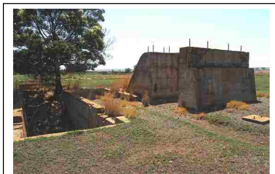
Fig. 7 Secondary crusher foundations.
