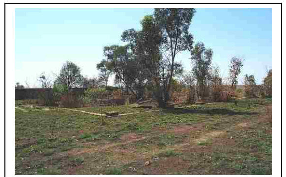
Fig. 6 Boiler plant external wall foundations.
