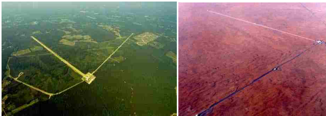
Figure 1-3: Aerial photos of the LIGO array. Left: The LIGO Livingston detector in Livingston, LA (LLO). Right: The LIGO Hanford detectors in Hanford, WA (LHO). The end station experiment buildings were positioned 4 km away from the corner station. The buildings at the mid-point of the LHO arms contain end mirrors for the 2 km gravitational wave detector. Identical buildings at LLO are empty.
