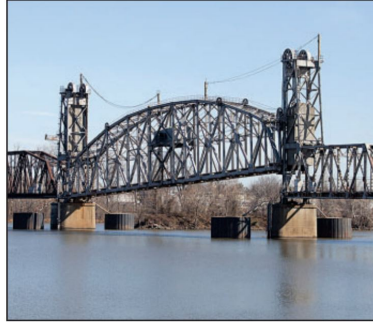
Figure 4.1. Arkansas and Missouri railroad bridge (McGeeny & Magsam, 2014)
