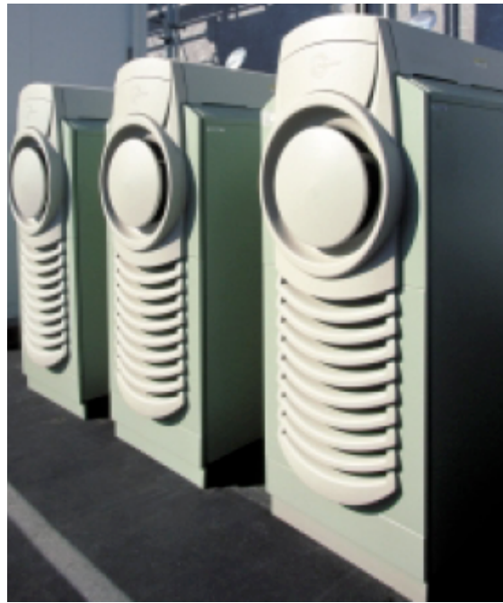
Figure 3.5 Three Capstone microturbines in operation [40]
