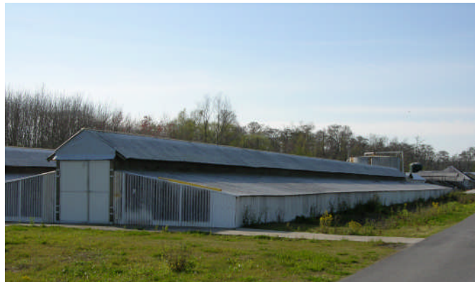
Figure 2. Buildings used for alligator ranching in Louisiana.
