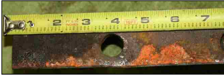
(a) Top of Channel
