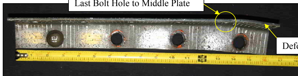
(b) East Channel Flange Rivet Surface
