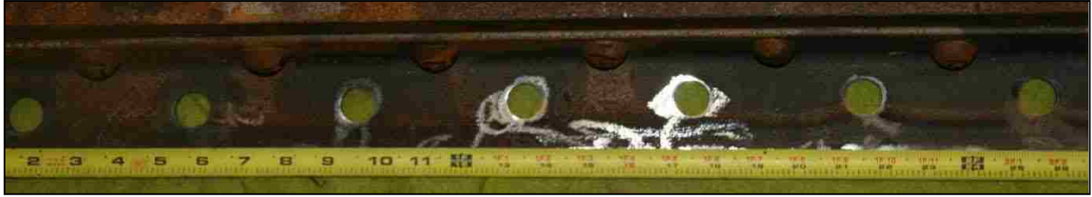
(a) East Channel Prior to Testing
