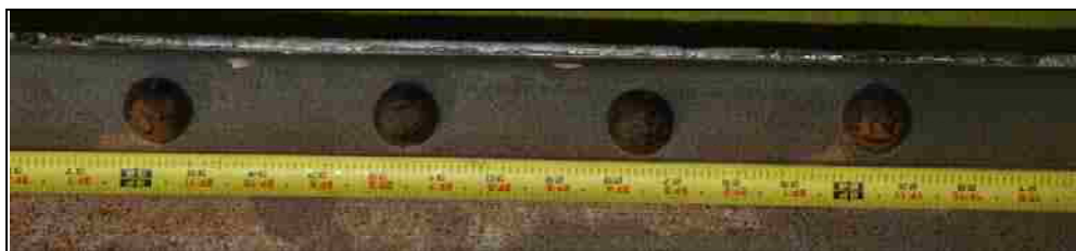
(a) West Channel Prior to Testing
