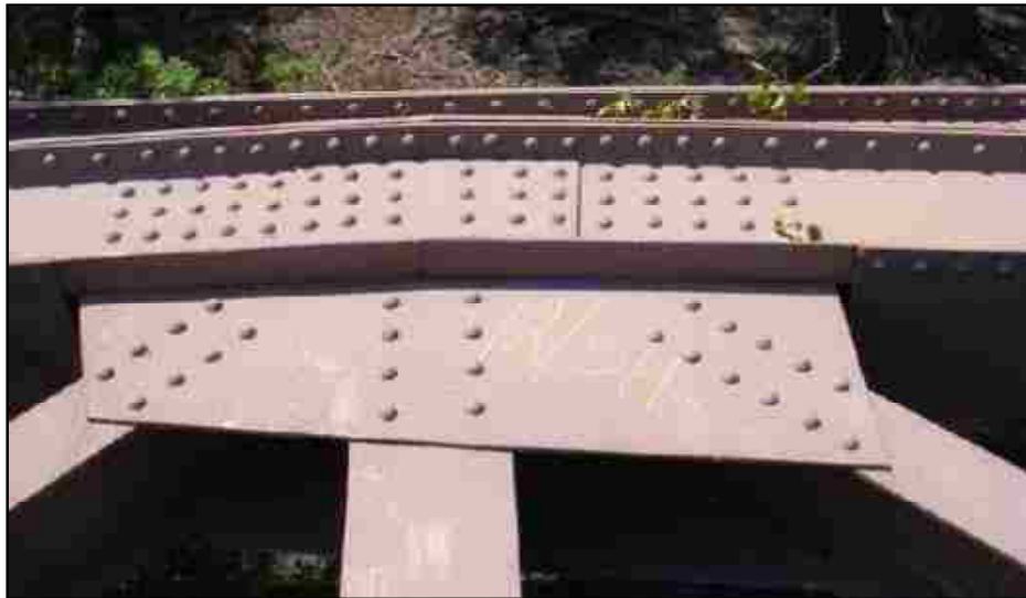
Figure 3.5 Joint U3 from Bridge 1
