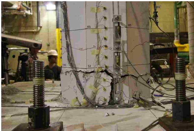
Figure 4-7: PreT-SS fully spalled.
