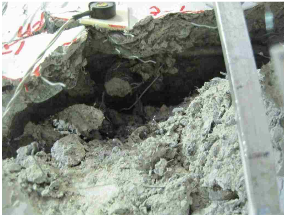
Figure C - 5: Fracture of longitudinal reinforcement, cycle 8-1.
