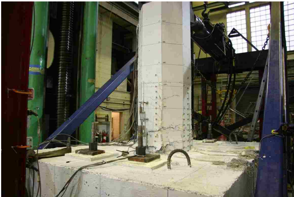
Figure C - 3: Column fully spalled, cycle 9-1.
