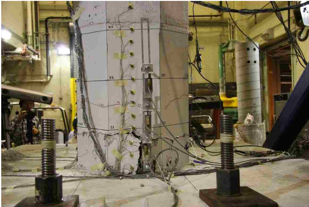
Figure C - 10: Column fully spalled, cycle 9-1.
