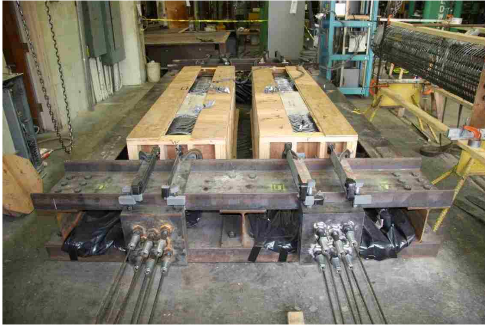
Figure 2-14: Strands stressed inside the HyFRC shells, ready for casting.
