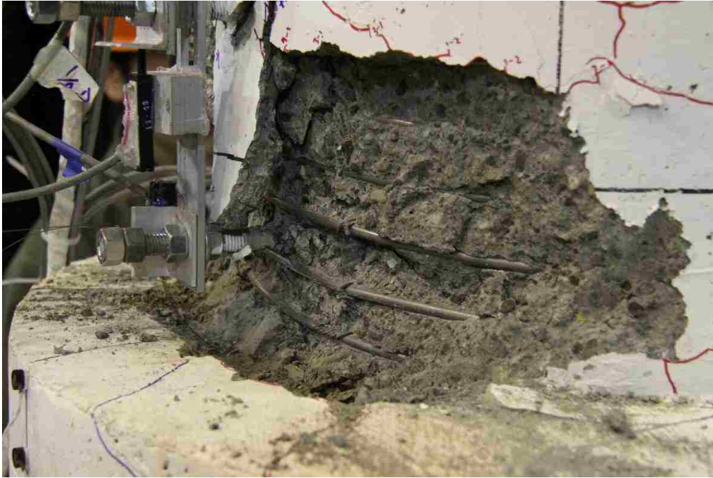
Figure C-0-4. DS-1 – First noticeable bar buckling in the column in Cycle 9-3 (6.90/-6.81 percent drift)
