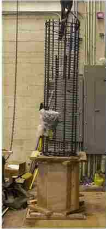
a). Column reinforcement
