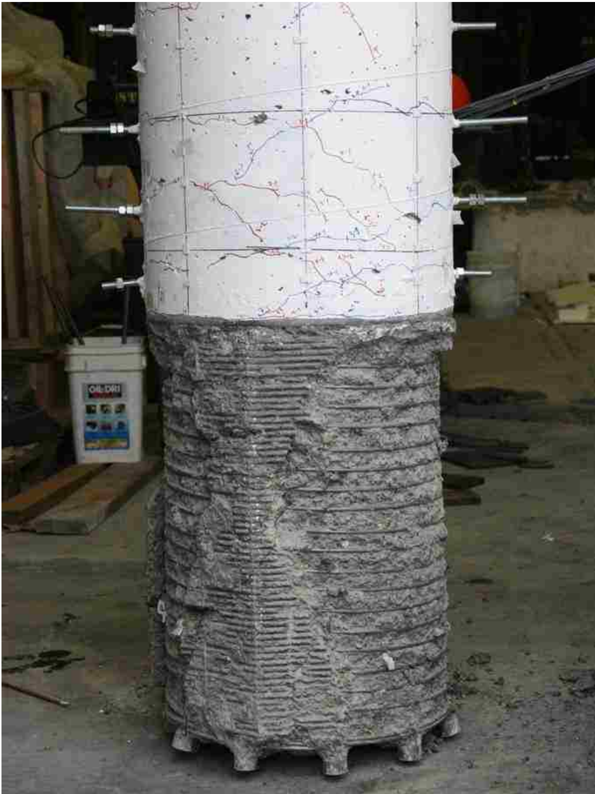
Figure C-0-13. DS-2 – Column damage after cyclic testing
