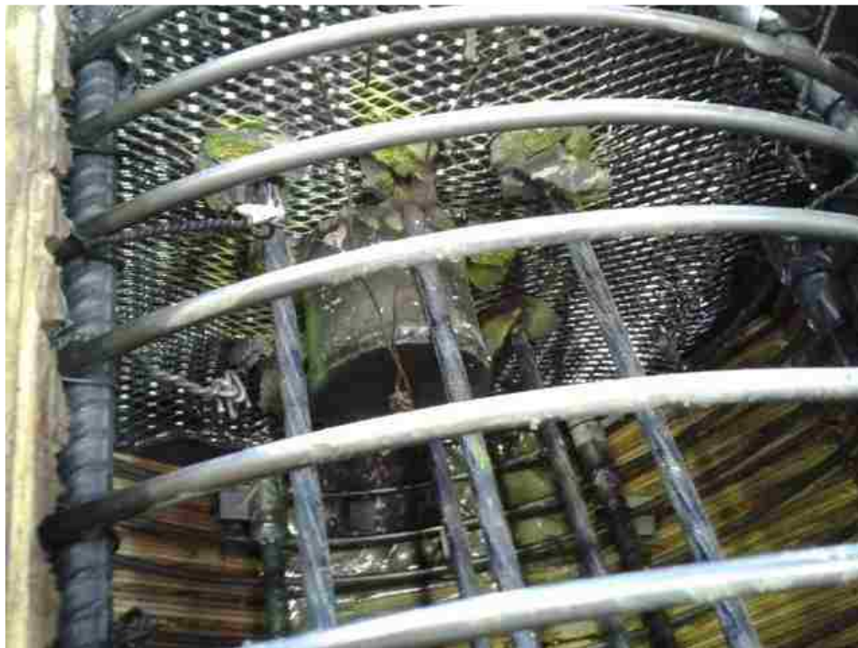
Figure D.3 Dividing mesh used to separate the HyFRC and conventional concrete pours. (Image after casting).
