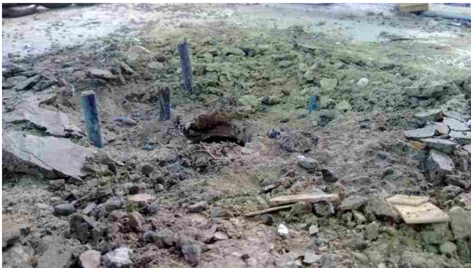
Figure C.7 Top of footing after testing.
