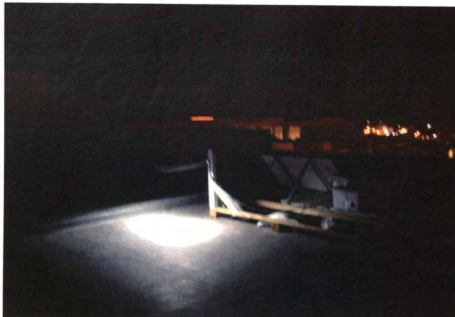
Close-up look at LED light in operation. The focused light provides pin point light directly beneath the lamp.
