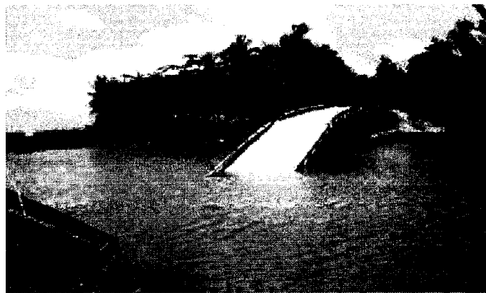
(b) Loss of support due to liquefaction, Rio Viscaya bridge, Costa Rica earthquake 1990
