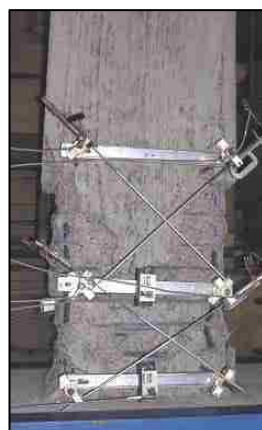
Figure 3.14 (F6 & F7) Longitudinal Bar Buckling and Crushing of Core Concrete
