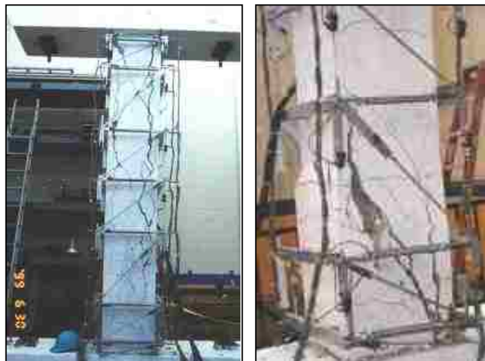
Figures 3.67 and 3.68 Widening and localization of shear cracks: experimental damage (Sezen 2002)
