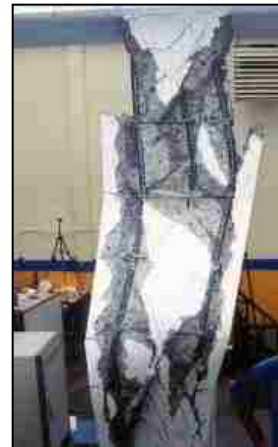
Figure 3.27 (S3.3) Longitudinal Bar Buckling
