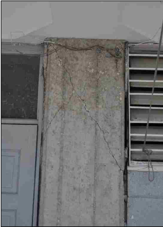
Figures 3.63 and 3.64 Shear cracking on side faces: earthquake damage (Sedra, et al. 2010)
