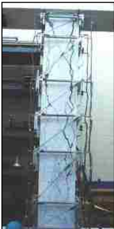
Figure 3.24 (S3.0 & S3.1) Widening and Localization of Shear Cracking and Longitudinal Cracking on Side Face
