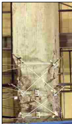
Figure 3.13 (F5) Concrete Spalling Exposing Longitudinal Steel
