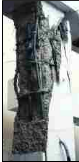
Figure 3.99 Crushing of core concrete: experimental damage (Sezen 2002)
