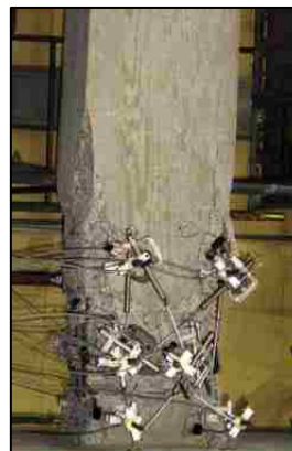
Figure 3.20 (F6 & F7) Longitudinal Bar Buckling and Crushing of Core Concrete
