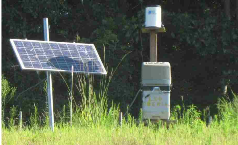
Figure A.5. ISCO auto-sampler unit with energy source and rain gauge.
