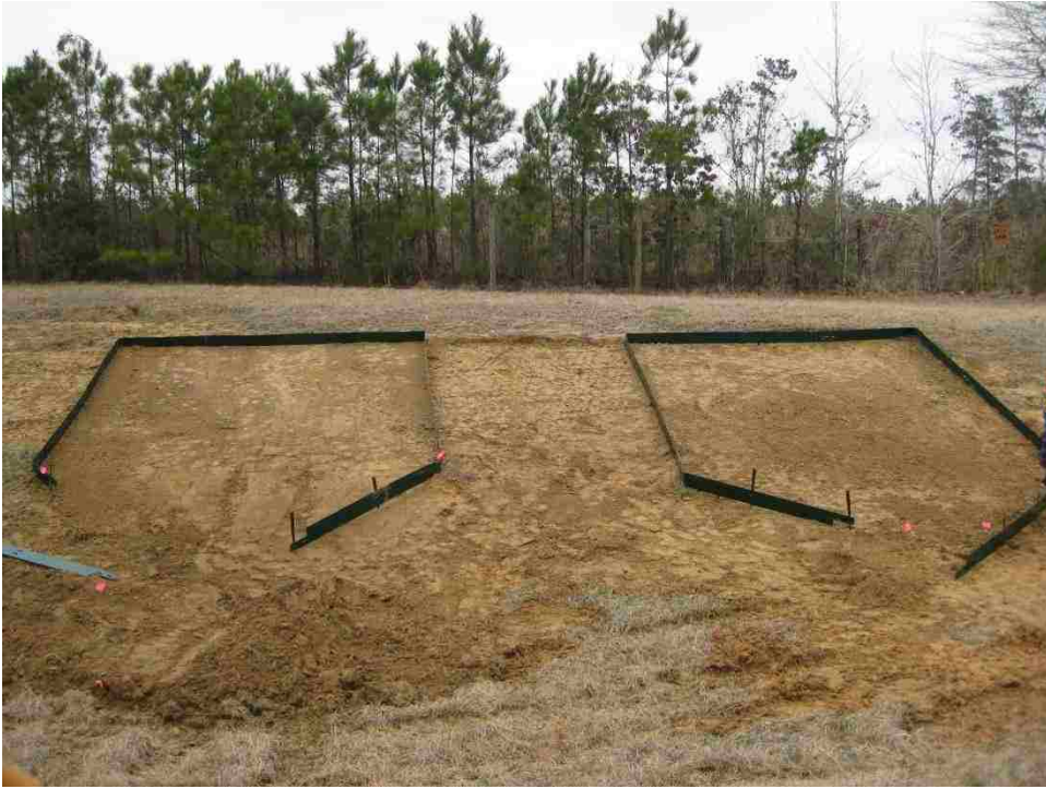
Figure A.3. Adding heavy steel edging.
