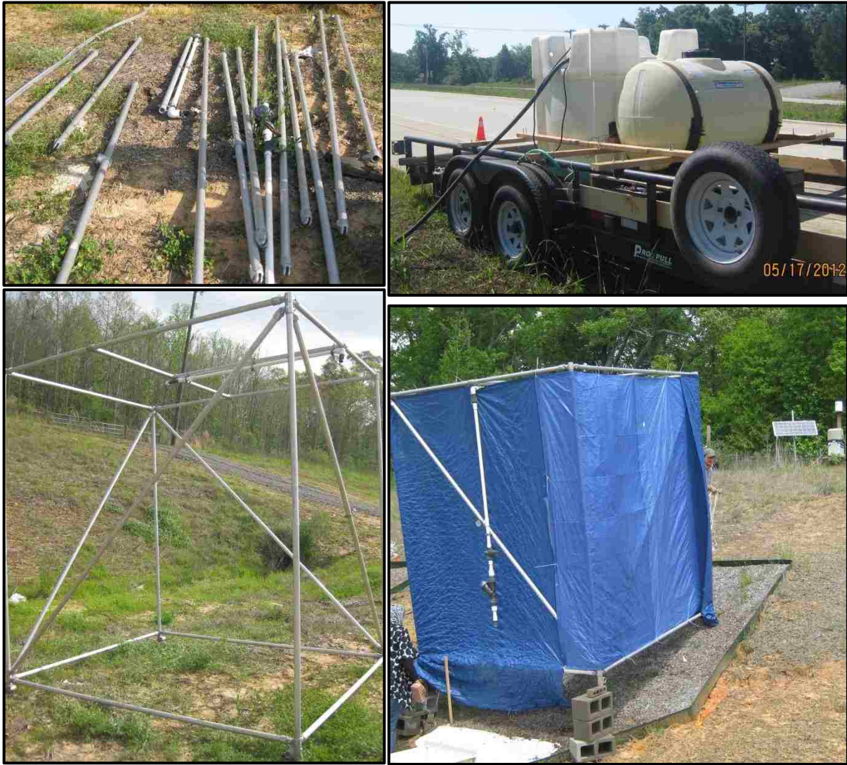
Figure 7.2. Rainfall simulator installation and application in the study sites in Louisiana, USA.
