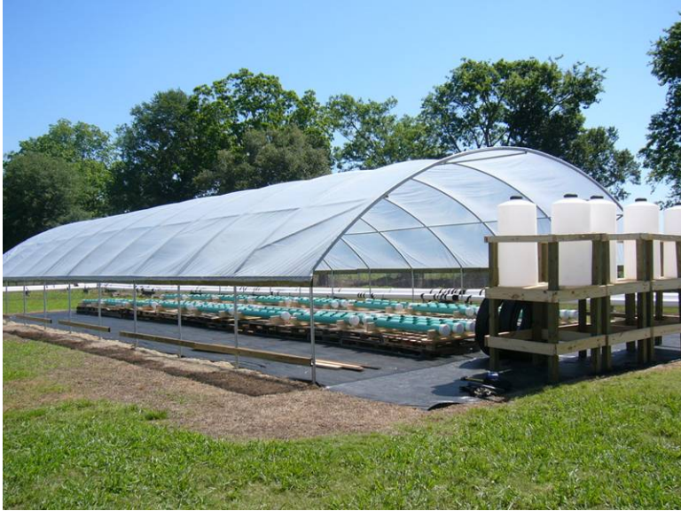
Figure A-3. Before end walls were constructed
