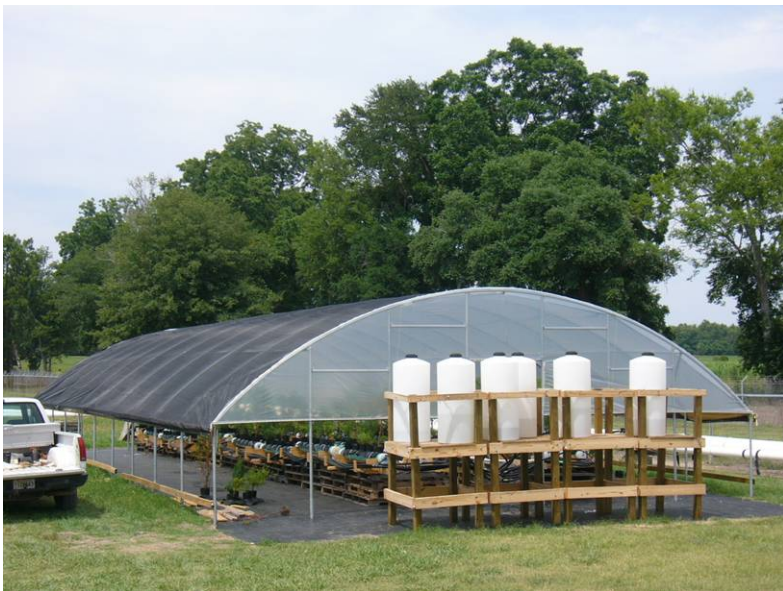
Figure A-4. After construction of end walls
