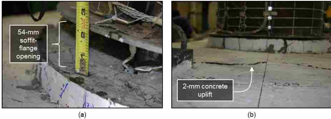
Figure 5.47: WRCUB (a) Soffit-flange opening at first bar fracture, and (b) South concrete uplift at 10.53% drift North
