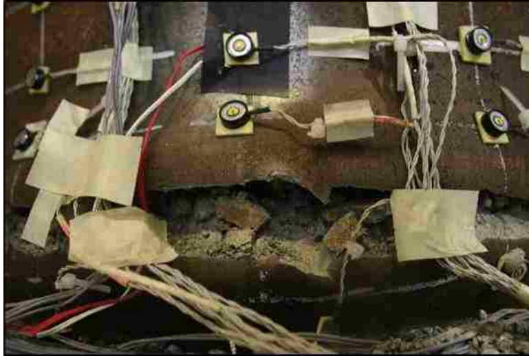
Figure 5.12: EMB80 tear propagation on North side of column at 8.54% drift
