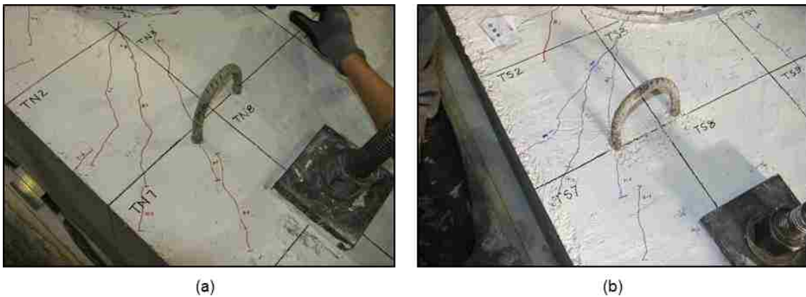
Figure 5.23: WRC cap beam cracking during the 11 th cycle level (a) North side of specimen, (b) South side of specimen
