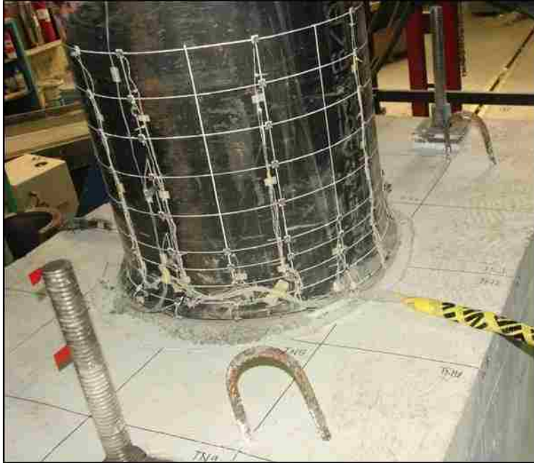
Figure 5.73: EMB96 Specimen damage at termination of test
