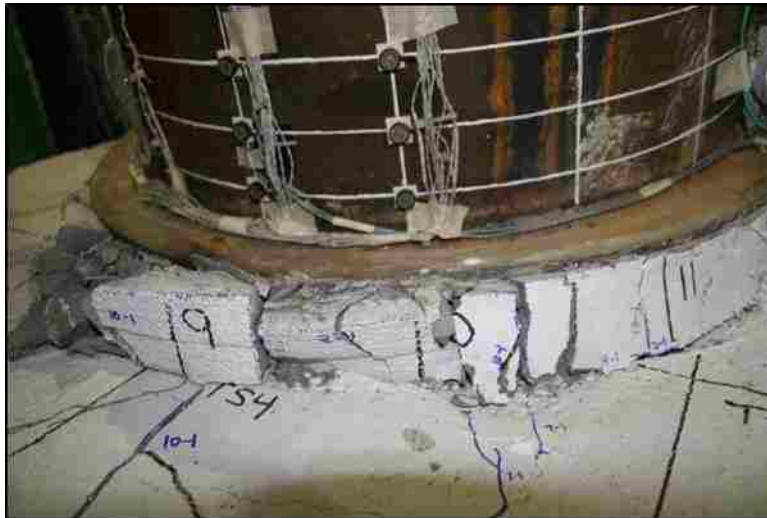
Figure 5.34: WRC South soffit damage at 11.47% drift South
