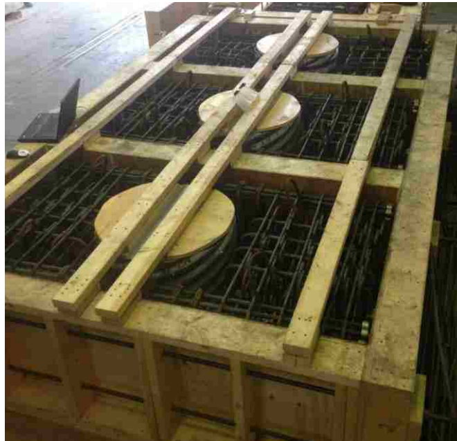
Figure 4.7: Cap Beam Reinforcing and Formwork
