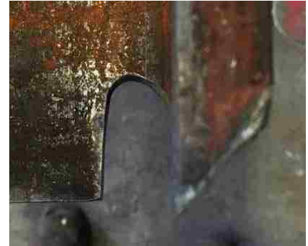
Figure 3.25: Completed weld access hole.
