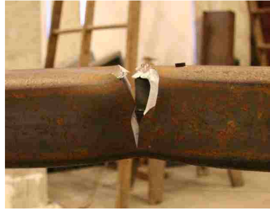
Figure 4.83: N brace \frac{3}{4} tear at -3.3% drift (B3-BT).
