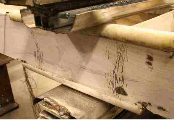
Figure 4.65: Beam yielding at 0.83% drift (Y1-OF).
