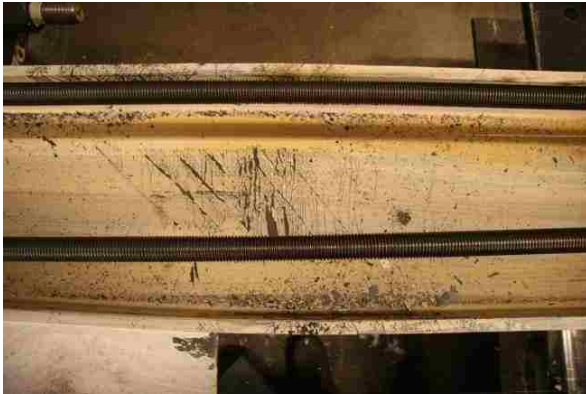
Figure 4.45: Initial col. local buckling at 2.2% drift (LB1-OF/IF).
