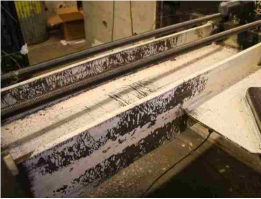
Figure 4.76: N col. severe yielding at 2.8% drift (Y3-PH).
