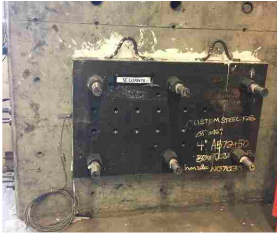
Figure 3.7: Interface plate attached to strong wall.
