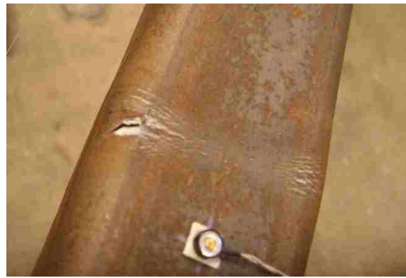
Figure 4.81: N brace crack/striations at -3.3% drift.
