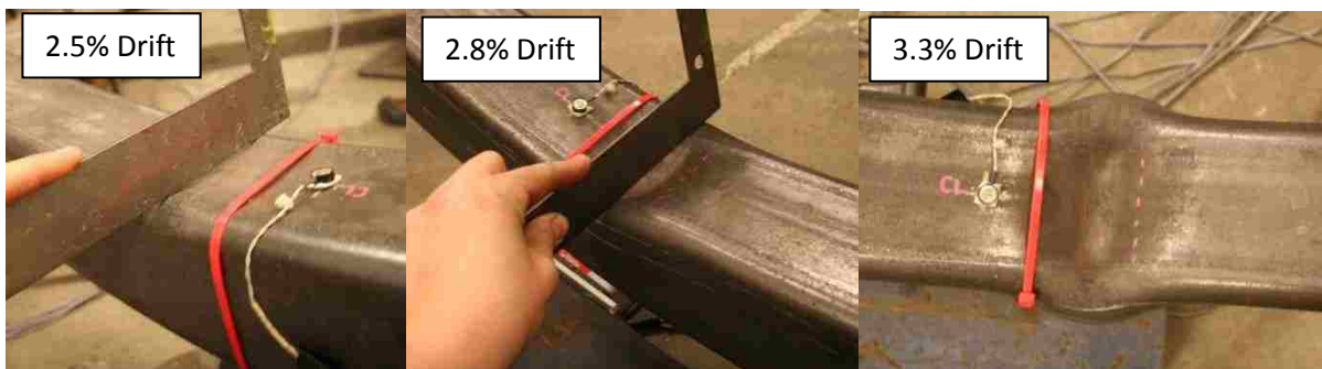
Figure 4.47: Progression of local cupping in S brace (B3-PH).
