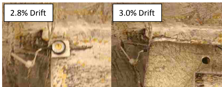
Figure 4.20: Crack propagation in S mid-span gusset-to-beam weld (WT1).
