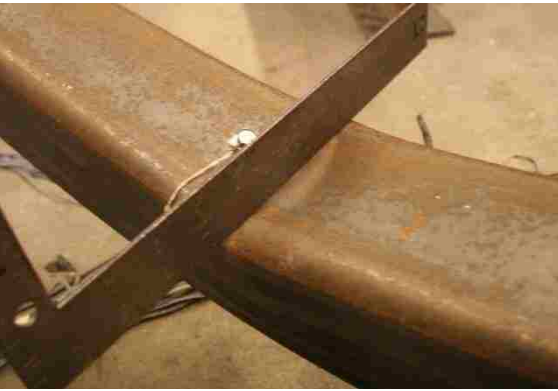
Figure 4.78: S brace cupping at 3.0% drift (B3-PH).
