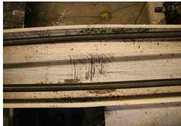
Figure 4.75: Initial N col. local buckling at 2.2% drift (LB1-OF/IF).
