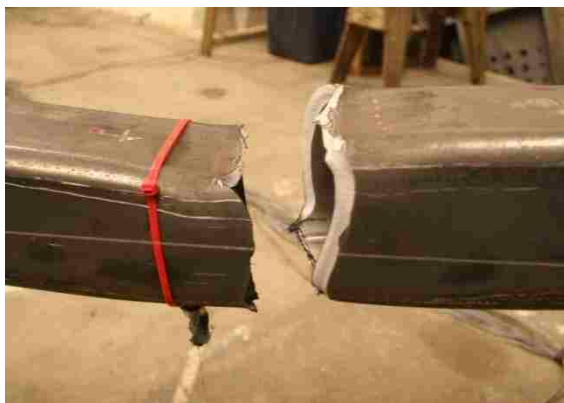
Figure 4.52: S brace fracture 1 st cycle at 3.3% drift (B4-BF).
