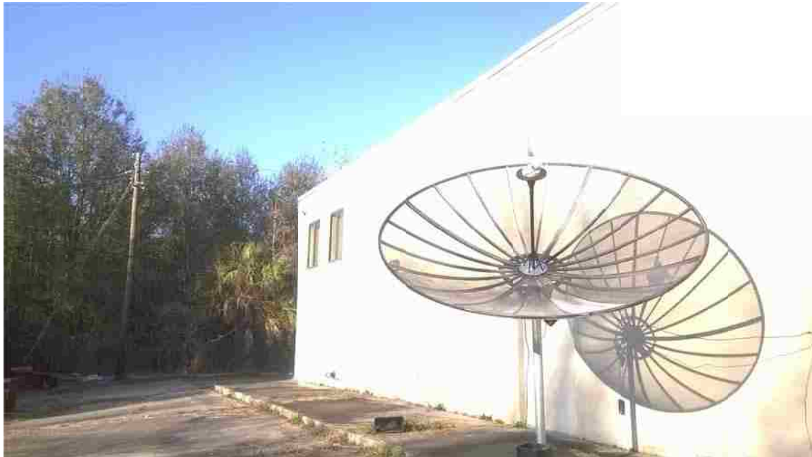
Figure 5-4: My 10' NOAAPORT dish. Due to large download sizes, going forward input data will be captured from the NOAAPORT satellite broadcast network.
