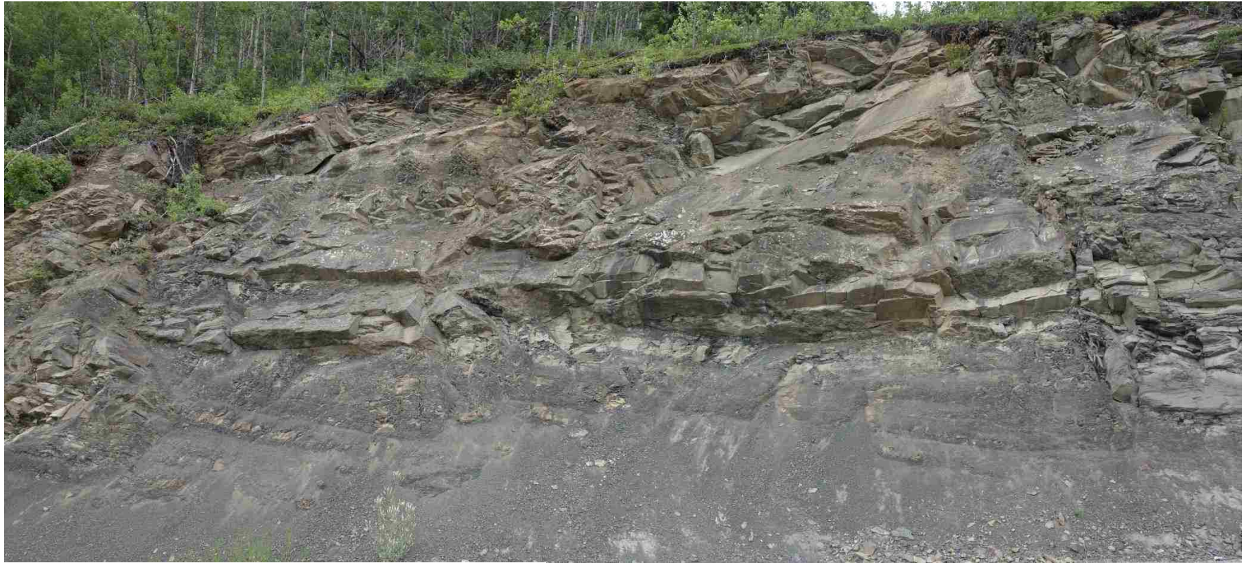
Figure 2.13 (above): Chickaloon formation at Milepost 87 along Glenn Highway. This site has soft sedimentary rock overridden by hard mafic sills causing differential erosion resulting in overhangs within the slope.
