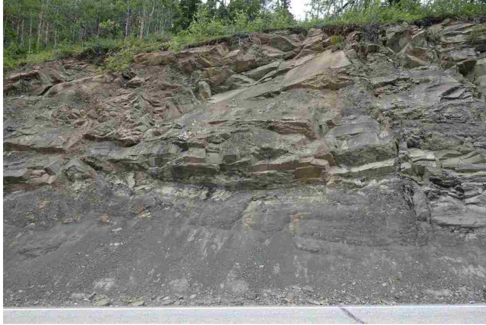
Figure 2.10: Carbonous siltstones overridden by a sill. The siltstones are a weaker material and therefore erode faster than the sill causing overhangs within the sill. To the right a fault can be seen offsetting these strata. These faults can be seen throughout the Chickaloon formation.
