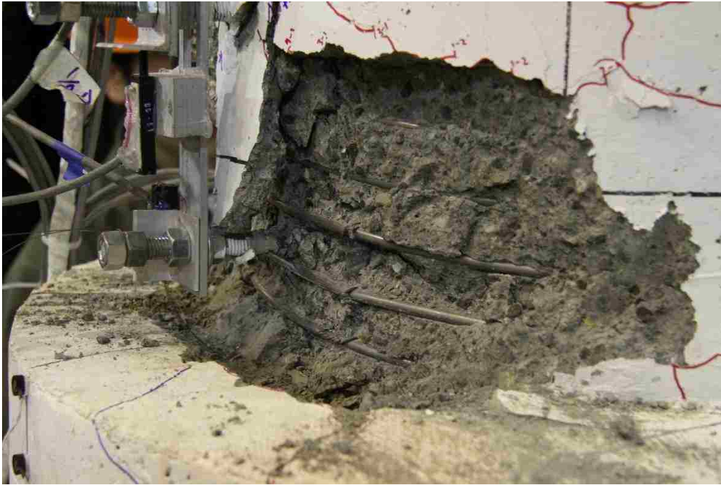
Figure C-0-4. DS-1 – First noticeable bar buckling in the column at 6.90/-6.81 percent drift
