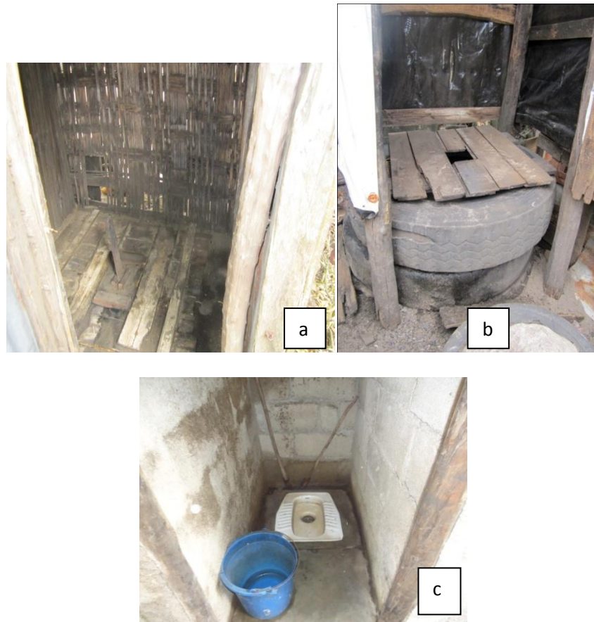
Figure 5: Common forms of on-site sanitation facilities found in Tamatave, Madagascar. a) Simple pit latrine (picture taken by the D. Brad Akers); b) simple pit latrine lined with a metal drum (picture taken by the author); c) pour-flush latrine (picture taken the author)
