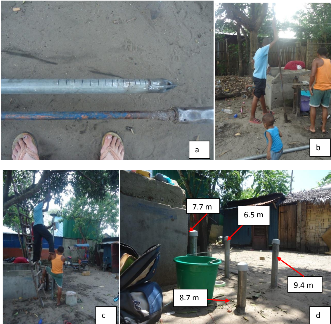
Figure 13: Materials and processes used to install the monitoring wells. (a) The GI outer casing (top) and agar(bottom) (picture taken by the author); (b) The technician's assistant drilling down near the water table (picture taken by the author); (c) The technician hammering the well into place (picture taken by the author); (d) Four completed monitoring wells with their corresponding depths noted (picture taken by the author).
