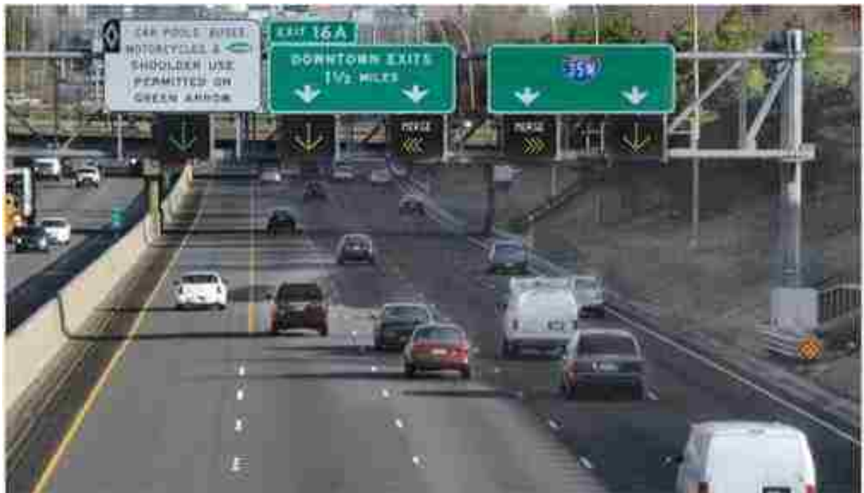
Figure 4. Intelligent lane control signals on I-35W
