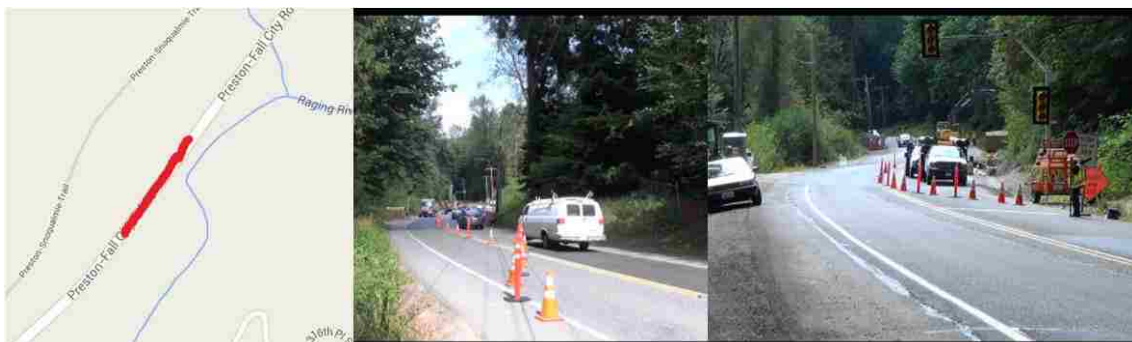
FIGURE A-4 Location and site photos for work zone #4
