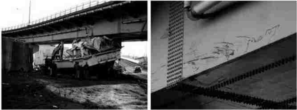
Figure 1-7: Fishing Boat Trapped Below Steel-Box-Girder Bridge (left) (Kriebel), Causing only Superficial Damage (right) (Robertson) (with permission from ASCE)
