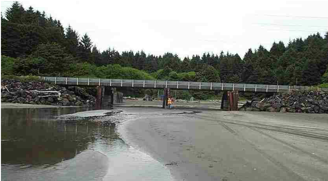
Figure 6-2: Wreck Creek Bridge (WSDOT, 2003)
