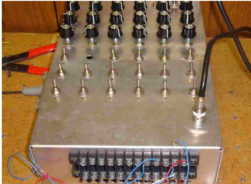
Figure 7-7: The switchbox contains the mechanical switches, input signal from the function generator, and the output of each switch is wired to a liquid crystal cell.
