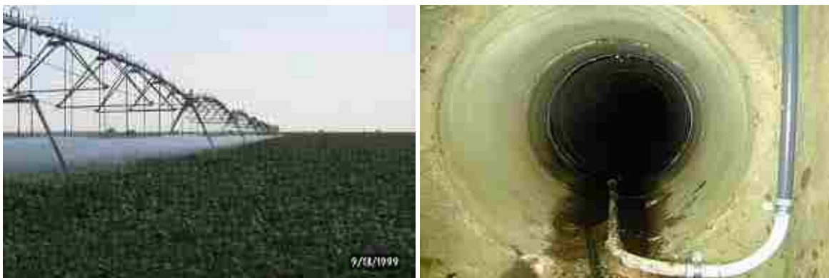
(a) Water pipeline for farming area
