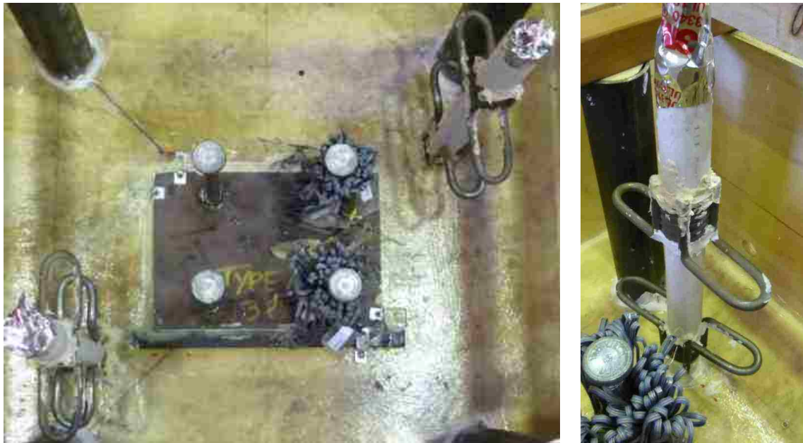
Figure 6.2.4.1: Lifting rods and their coil inserts
