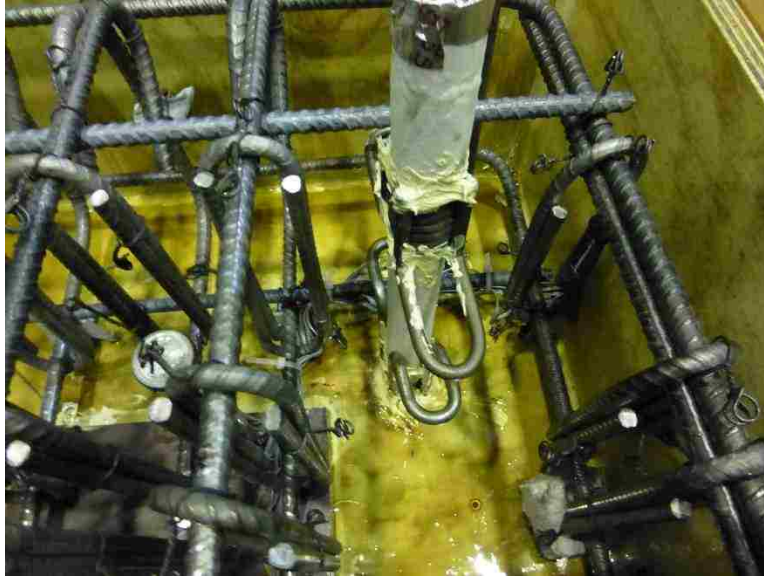
Figure 6.2.5.4: Strain gauge wires secured to the nearest rebar
