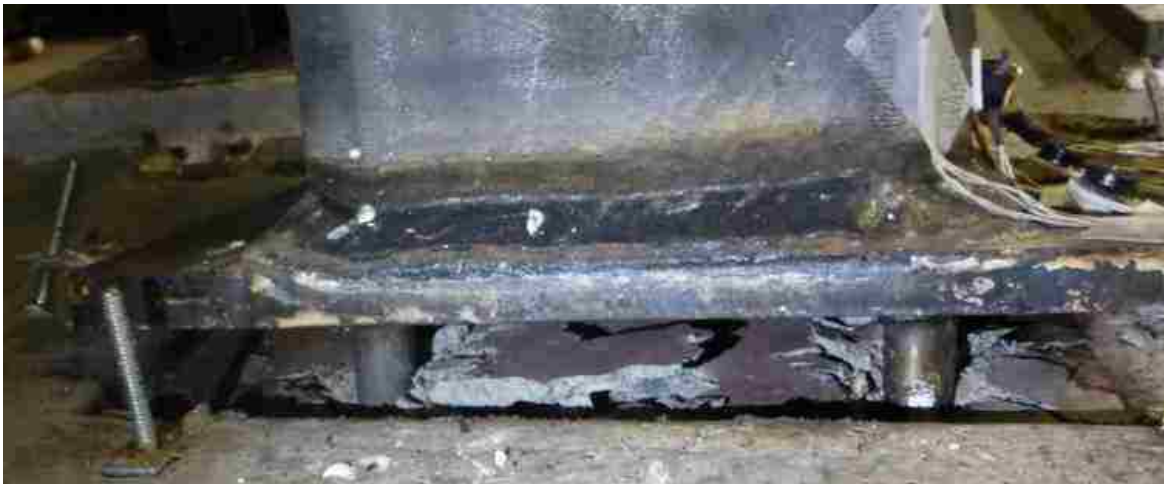
Figure 6.5.3.5: Concrete profile around the studs after failure (Specimen 2-2-0.92)
