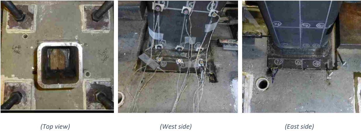
Figure 6.5.2.3: Crack patterns near embed plates after failure (Specimen 4-0-0.92)
