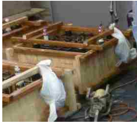
Figure 6.2.5.5: Strain gauge wires protected for casting process
