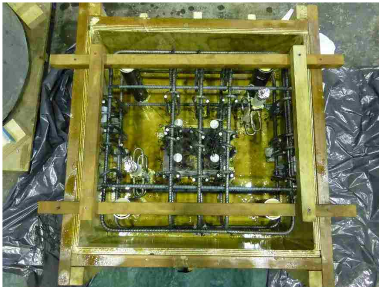
Figure 6.2.5.3: Rebar cage and steel pipes secured in place
