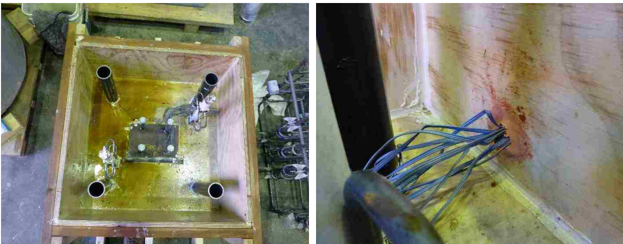
Figure 6.2.5.1: Strain gauge wires going out of the formwork
