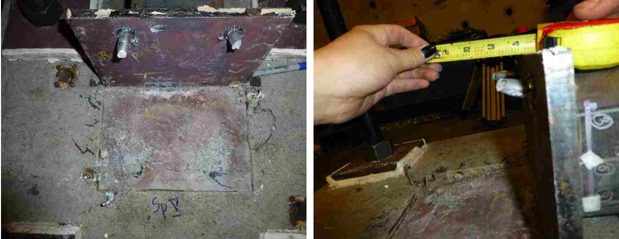
Figure 6.5.1.5: Specimen 2-0-0.92's sheared studs and local concrete crack profile
