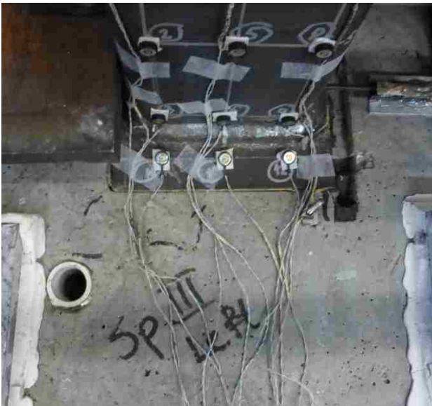
Figure 6.5.5.2.a: Concrete crack pattern at P=60 kips (Specimen 2-2-0.50)
