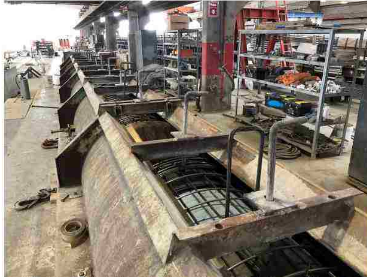
Figure 7-10. Column formwork ready to be line-cast at Concrete Technology Corporation
