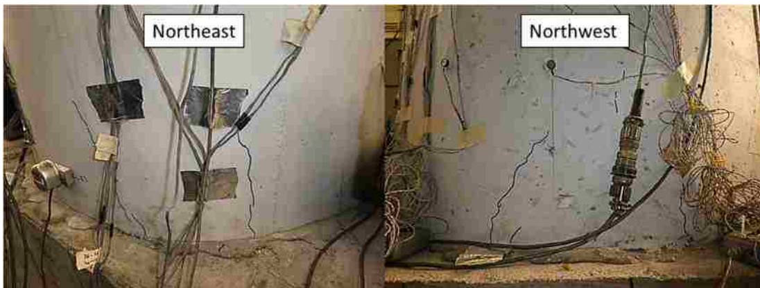
Figure 8-4. Short, fine cracks, Series 2
