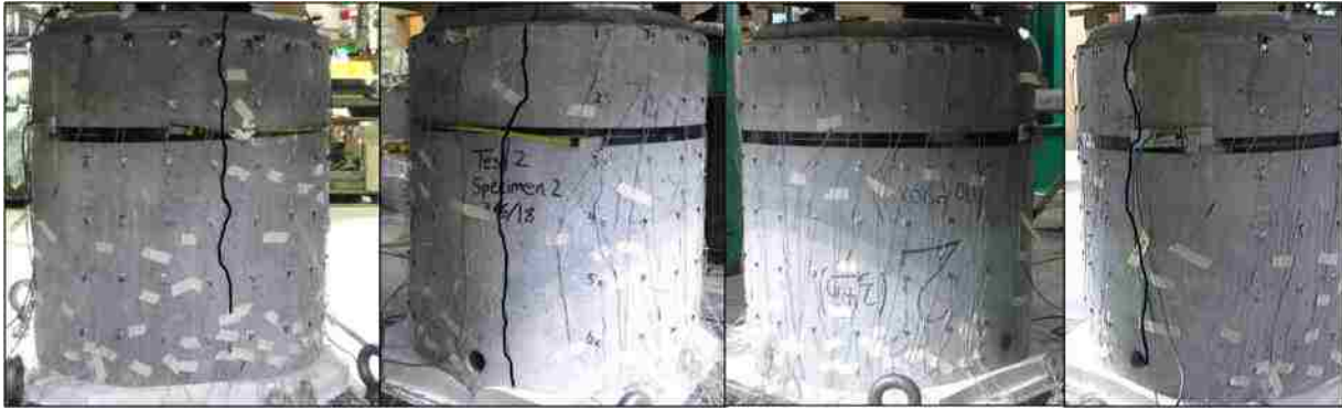
Figure 5-7. Crack formation at peak load for Test ep0-1 (L-R: N-SW-SE-NE)
