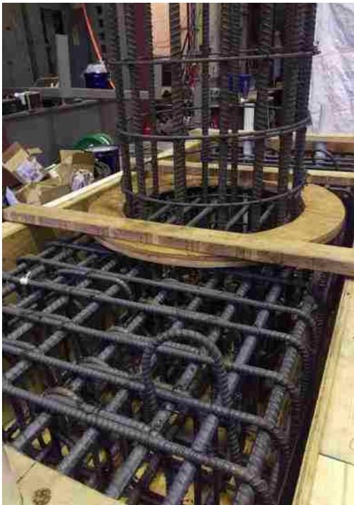
Figure 7-16. Cap beam and plug reinforcement in formwork before casting
