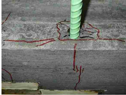
Figure 6.3. Typical structural damage observed during bond curb experiments.
