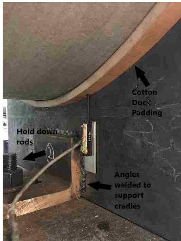
Figure 3-21. Support cradle arrangement
