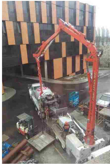
Figure 3-13. Concrete pump truck used for fill concrete
