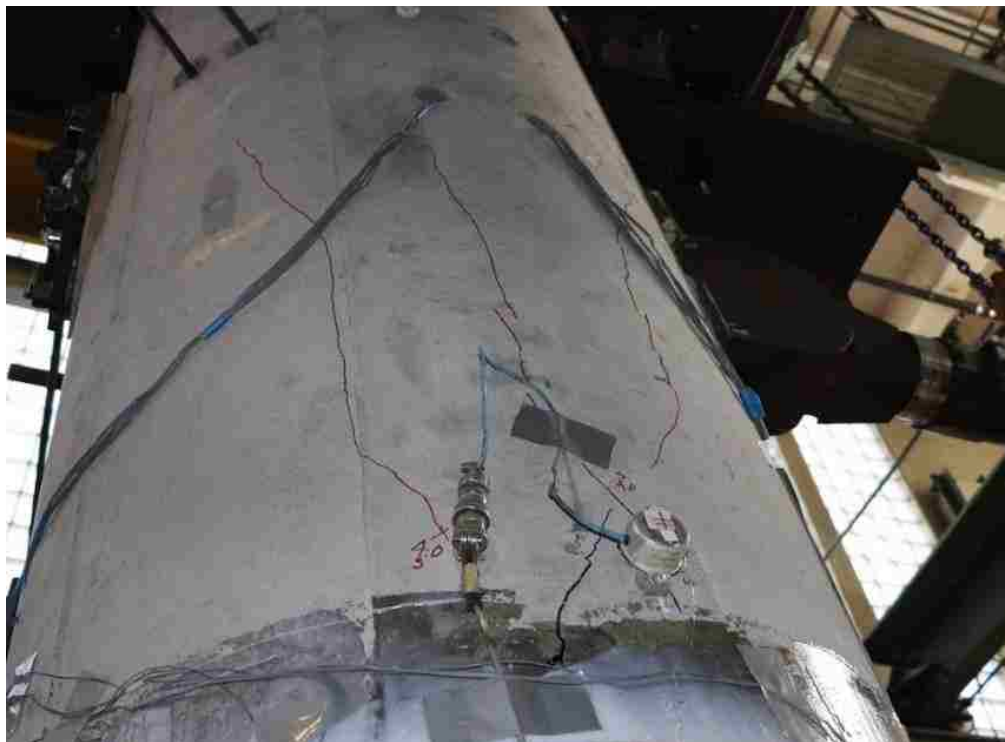
Figure 7-8. Progressive cracking above fiber on Series 8 (+4.71%, -5.49%)
