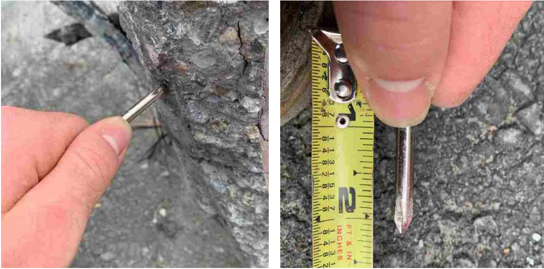
Figure 7-23. Measuring of the strand slip
