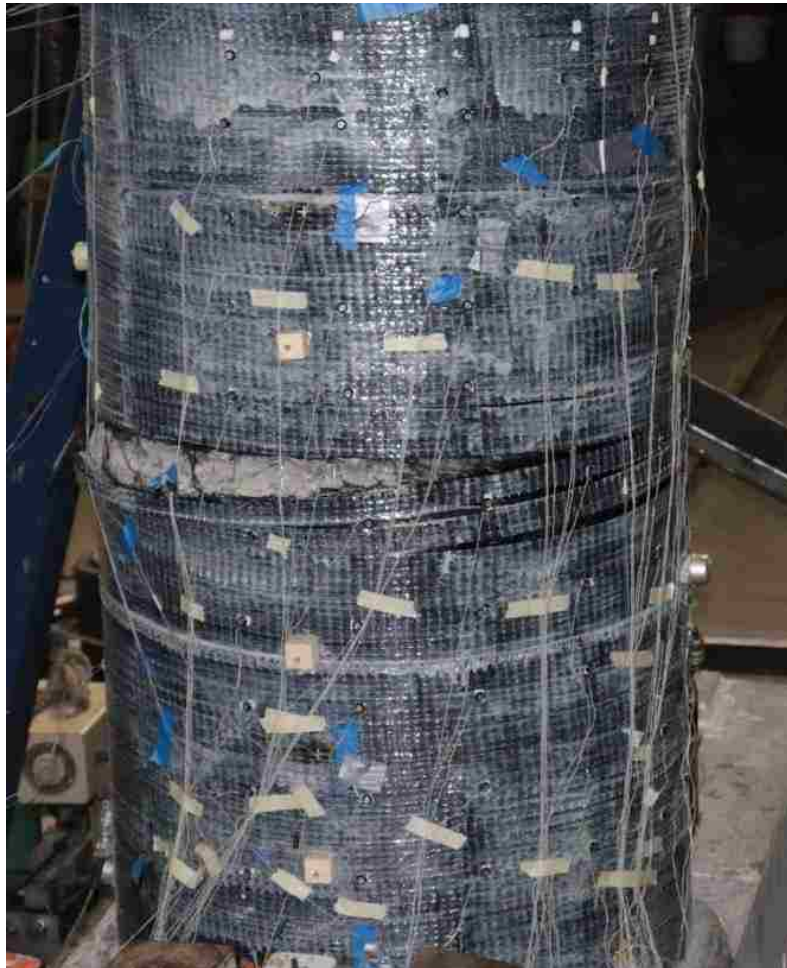
Figure 7-14. Fiber rupture on north face during Series 11
