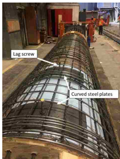
Figure 3-11. Hold-down plates used for sonotube during casting
