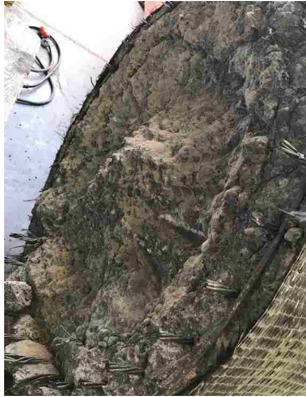
Figure 7-19. Top segment of specimen after detachment from plug connection to cap beam
