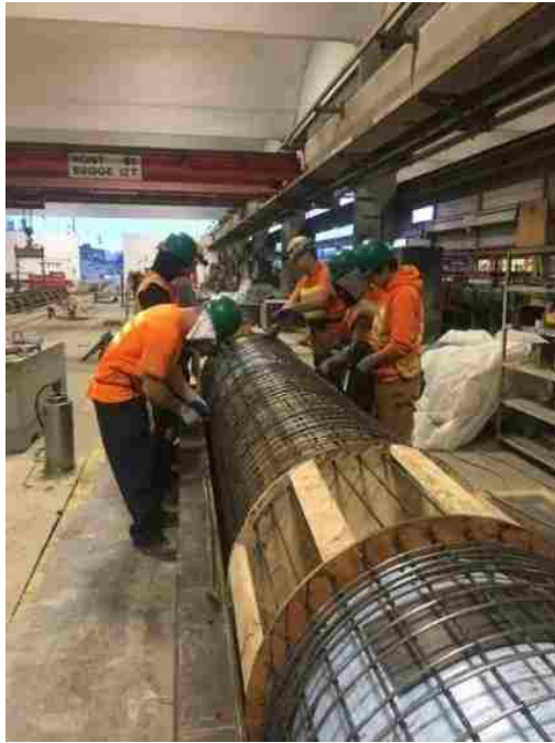
Figure 3-8. Pile-column reinforcement being prepared for casting at Concrete Technology Corporation
