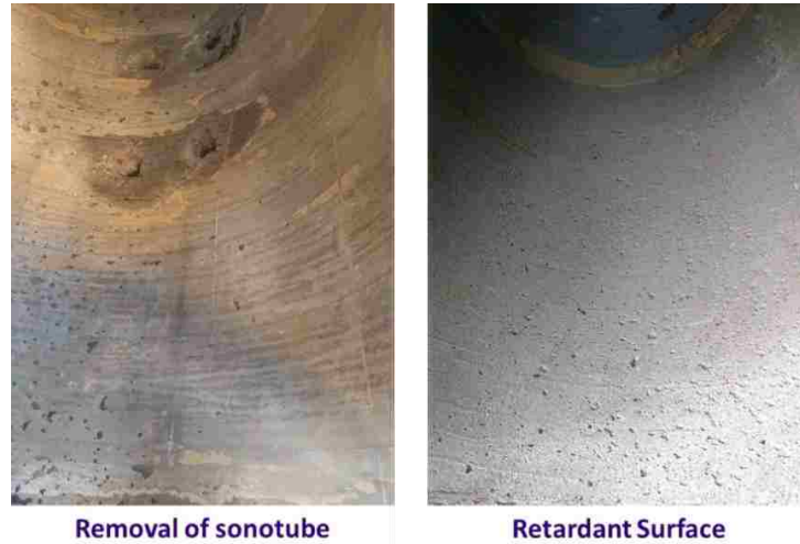
Figure 6-9. Comparison of surface roughness after removal of sonotube, with and without retardant
