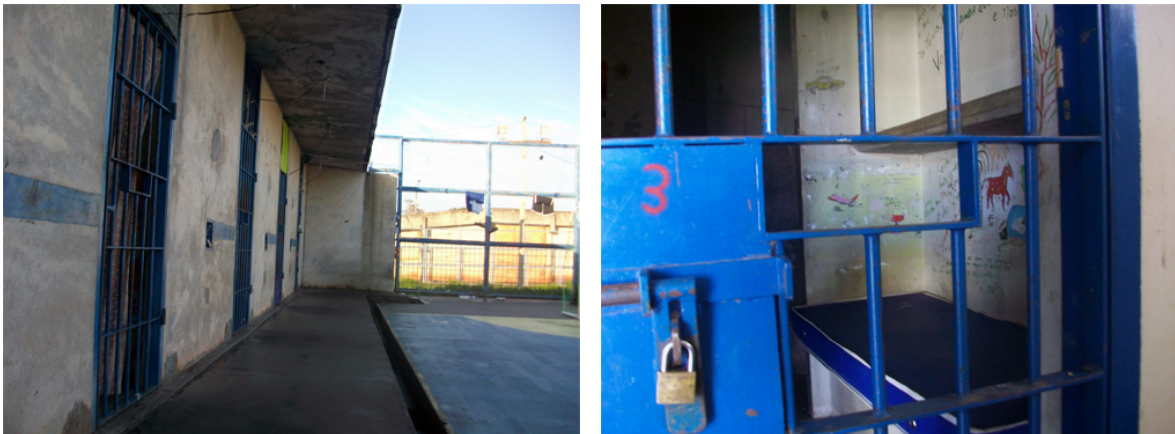
Figure S2. Partial architectural floor plan of typical general population cell courtyard in PTL (A). Photographs illustrating existing built conditions, 2013 (B).
